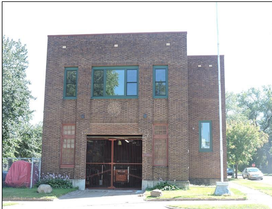
Figure 24. Engine House No. 24 at 1720 East Seventh Street, 2016
