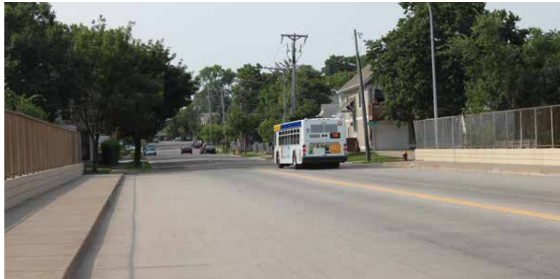
Figure 24: Earl Street bridge toward Indian Mounds Regional Park. The park is only \frac{1}{4} mile away, but is not visually connected to the bridge.
