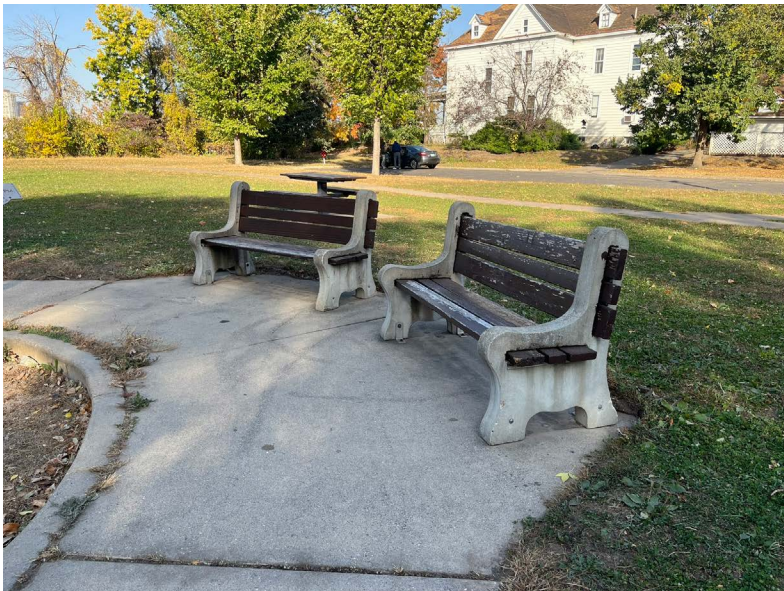
Benches in poor condition
