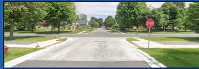
Along Wheelock Pkwy, Tabled Crossings Are Frequently Used along the Grand Round
