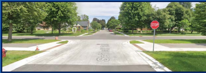
Along Wheelock Pkwy, Tabled Crossings Are Frequently Used along the Grand Round
