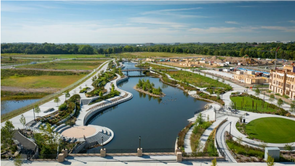
Figure 14: Highland Bridge Central Stormwater Feature
