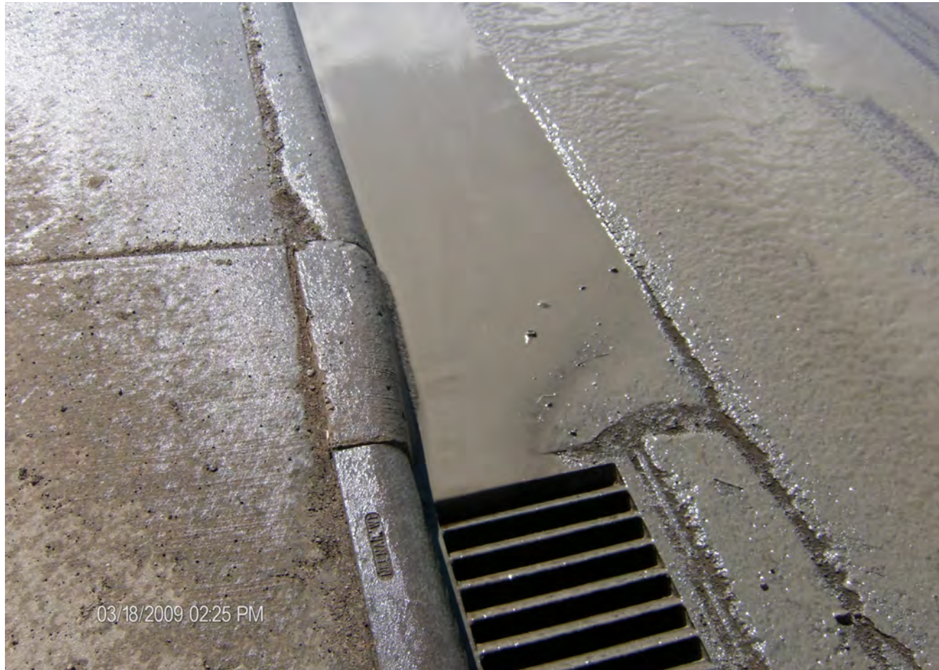
Discharge of Drilling Mud
