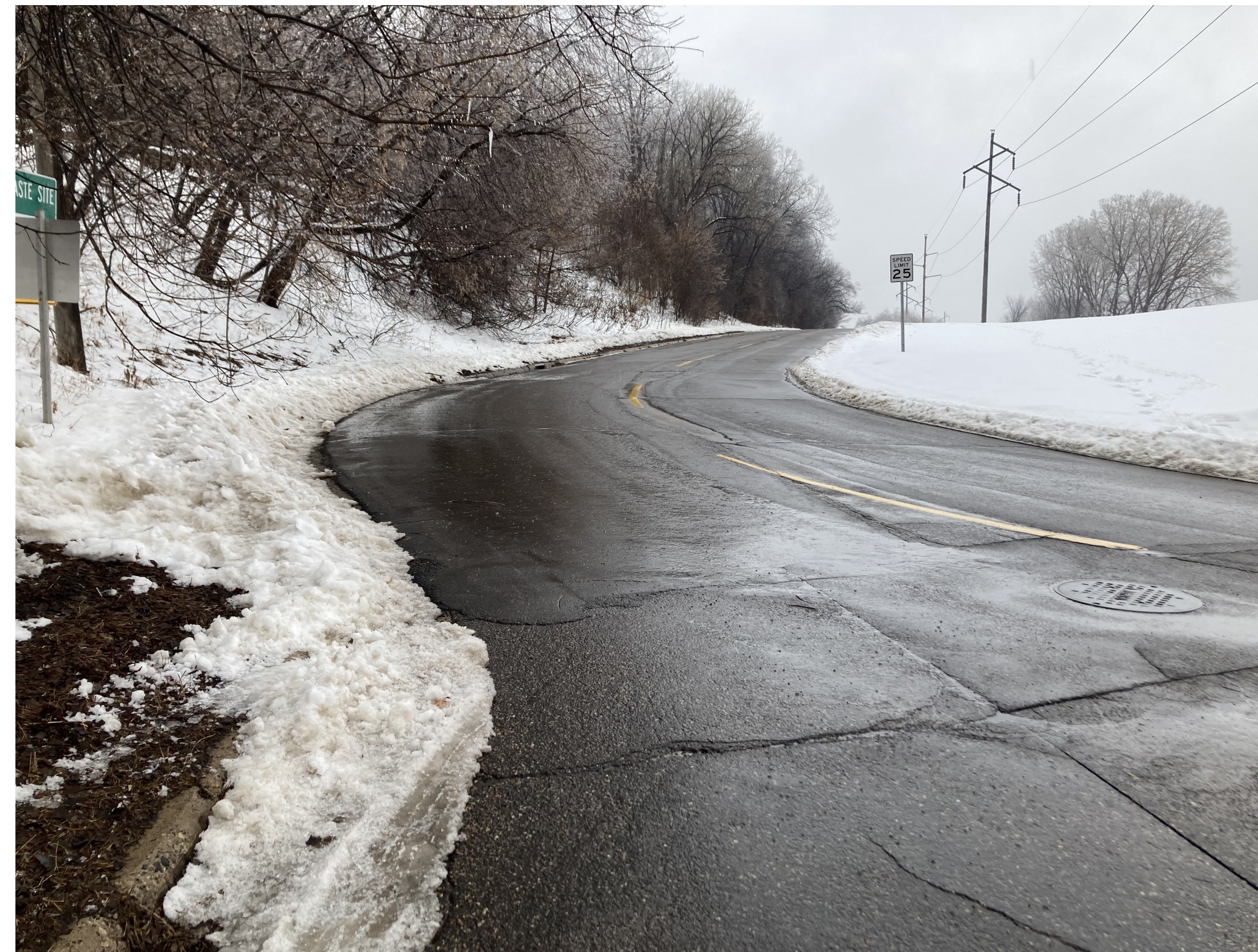
At the intersection of Behnill Road, Victoria Street and Pleasant Avenue. Looking east up Pleasant Avenue. Springs/seeps in Linwood Park create excess water along the steep north side, maintenance frequently addresses ice buildup in the winter months. Winter 2023.
