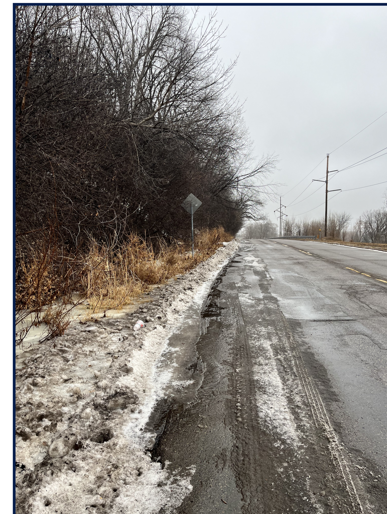
North side of Pleasant Avenue looking east. Snow and ice buildup on the north side. Winter 2024
