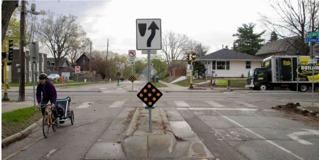
Motorists can only take a right off the 40 th Street Bicycle Boulevard at this traffic diverter located on Cedar Ave. Minneapolis, MN
