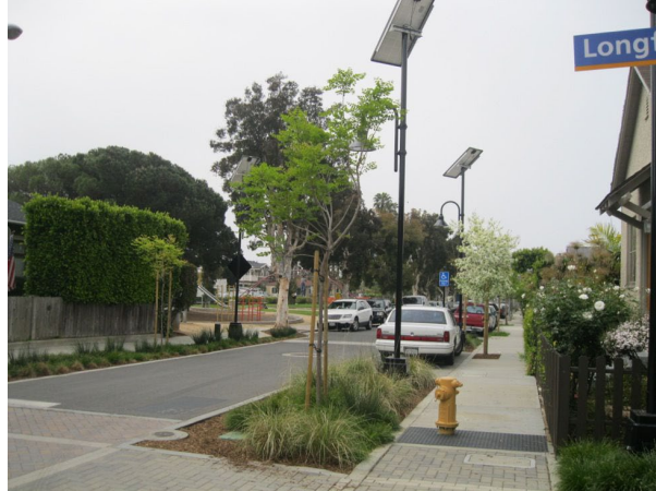
Curbless yield street with rain garden tree wells, solar street lights creates a more flexible street space. Source: NACTO.org
