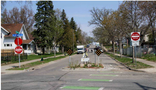
Half closures block one lane of vehicle travel, turning the bicycle boulevard into a one-way street for a short segment. Emerson Street Bicycle Boulevard and N 33 rd Ave. Minneapolis, MN
