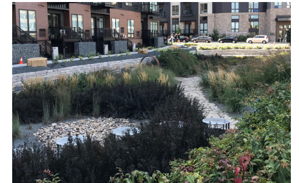
A : DISTRICT STORMWATER At key areas along district stormwater spine, the feature may widen to allow for additional rate and volume control, habitat, and recreation potential.
