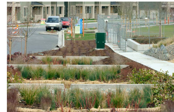
A : DISTRICT STORMWATER A green infrastructure spine will run between Howard Street and private light industrial parcels.
