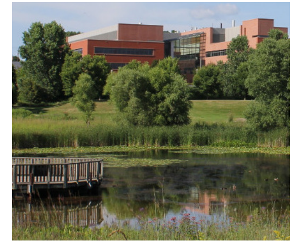
C : WETLANDS Three existing and two new wetland areas will provide flow and rate control for treated stormwater from the District Stormwater feature.
