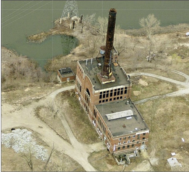
Figure 9. Island Station, looking south, 2012. (Bing)
