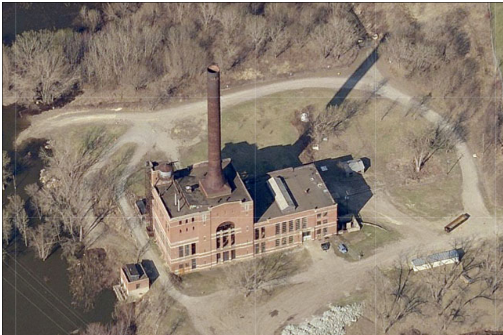
Figure 8. Island Station, looking northwest, 2012. (Bing)
