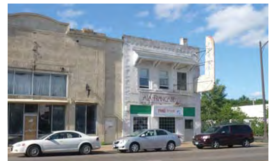
Former Victoria Theater and Ray-Bell Films buildings on University Ave.
