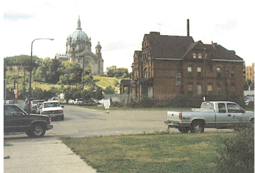
The Armstrong Quinlan house sits on the site of a proposed transit hub.
