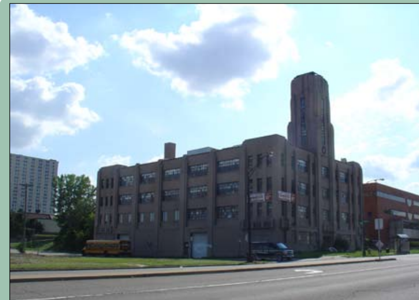
FIGURE 1.11 - The (former) Saint Paul Casket Company adds character and a sense of urban scale to the Avenue.
