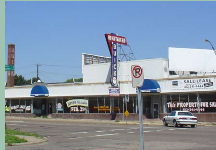
FIGURE 1.8 - Several auto-dealerships on the north side of University have recently vacated, providing opportunities for transit-supportive redevelopment.
