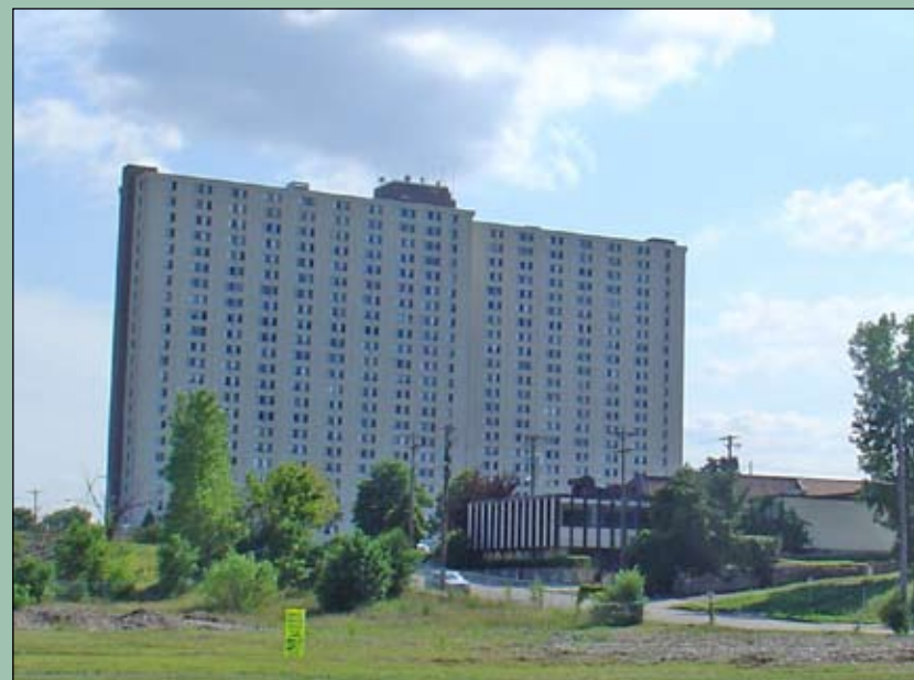
FIGURE 1.10 - Skyline Towers has parking and large vacant sites that front the south side of the Avenue, west of Lexington.
