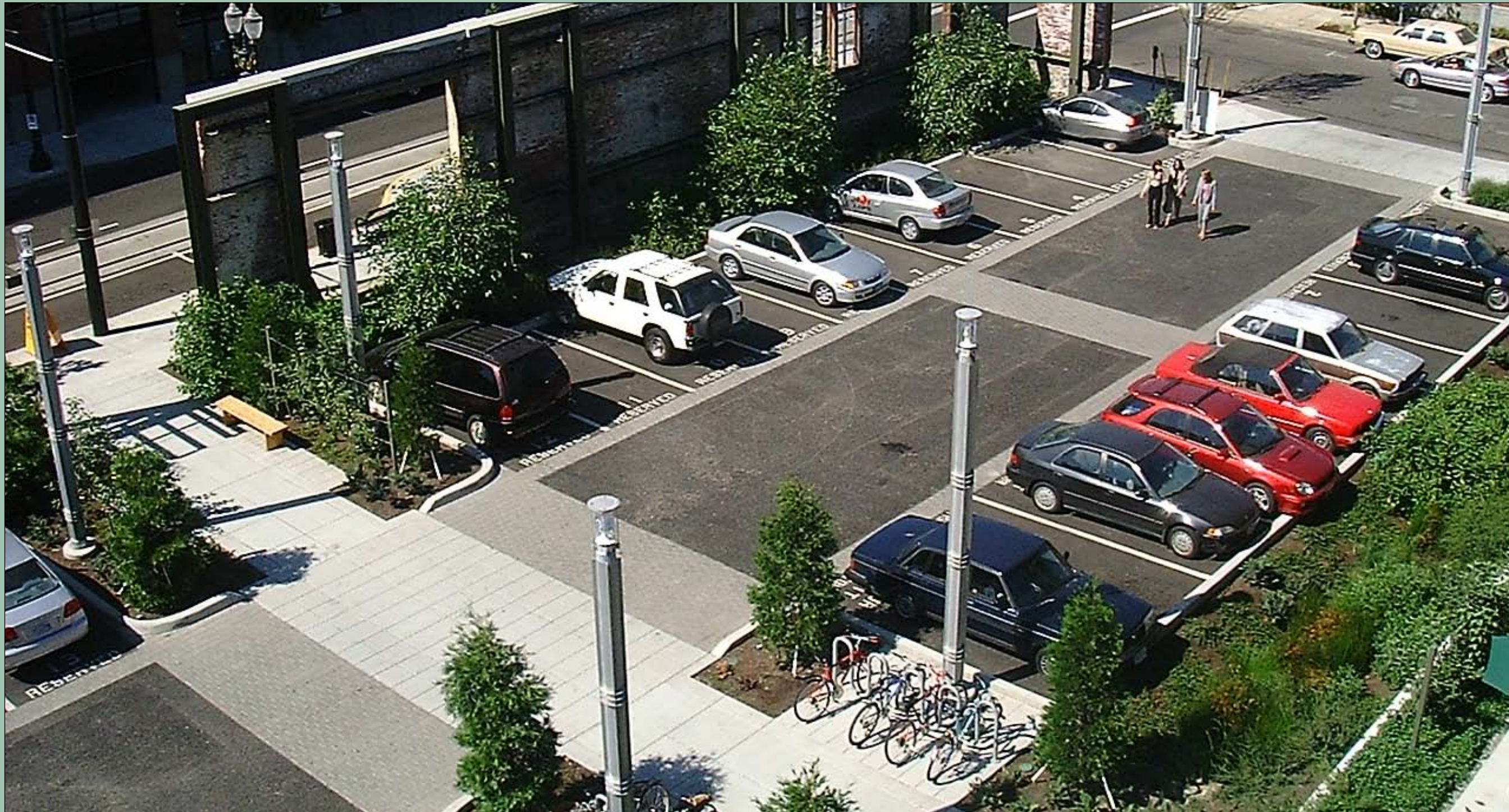
FIGURE 4.9 - A 56-foot wide surface parking lot in Portland, Oregon incorporates features such as permeable paving, integrated bike parking and pedestrian-scaled lighting. It is heavily landscaped and concealed from the street by an integrated former building facade.
