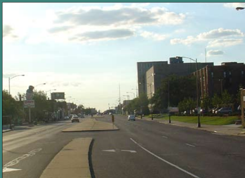
FIGURE 1.8 - Buildings currently lack a coherent relationship with the Avenue .
