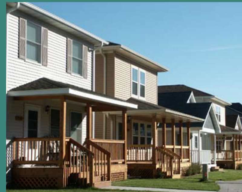
FIGURE 4.7 - Filling in the surface parking with similarly scaled housing such as these examples from Saint Paul will help restore and reinforce the neighborhood edge.
