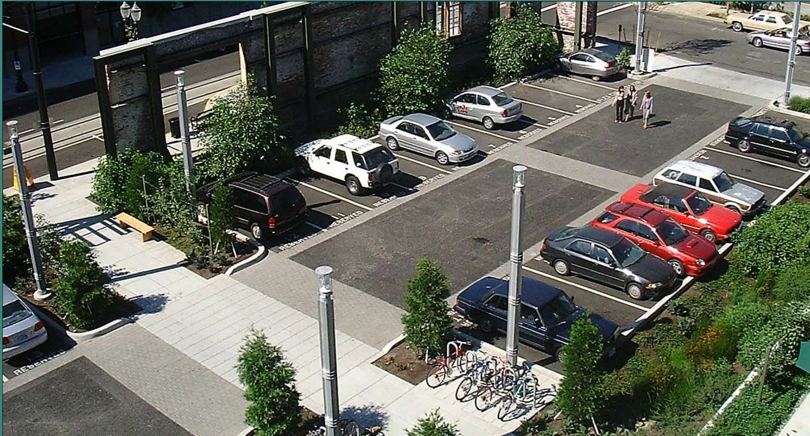
FIGURE 4.10 - A 56-foot wide surface parking lot in Portland, Oregon incorporates features such as permeable paving, integrated bike parking and pedestrian-scaled lighting. It is heavily landscaped and concealed from the street by an integrated former building facade.
