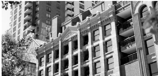
The development of Galtier Plaza incorporated the facade of a historic building into its design.
