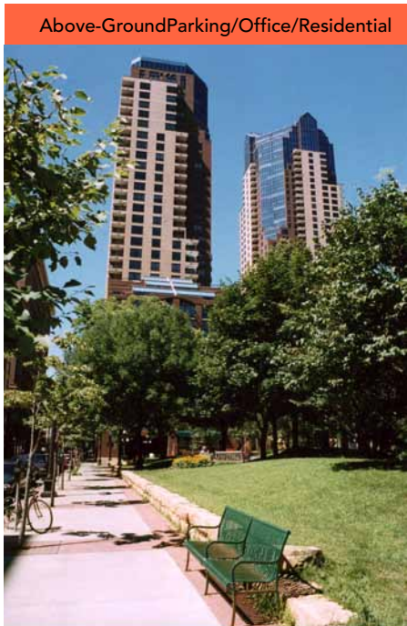
Galtier Towers (left), 172 6th Street East
