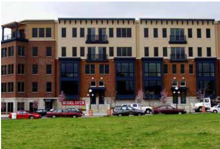
The Dakota, with 37 condominiums/townhouses, joins the Essex in providing the first new ownership housing in downtown in decades.
