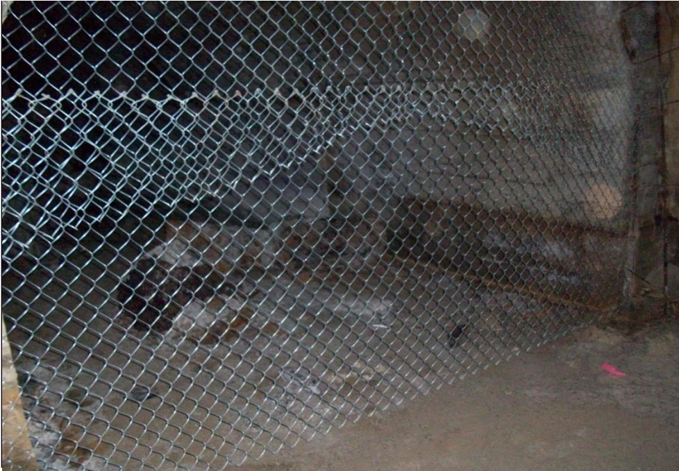
Chain Link Fencing Installation.
