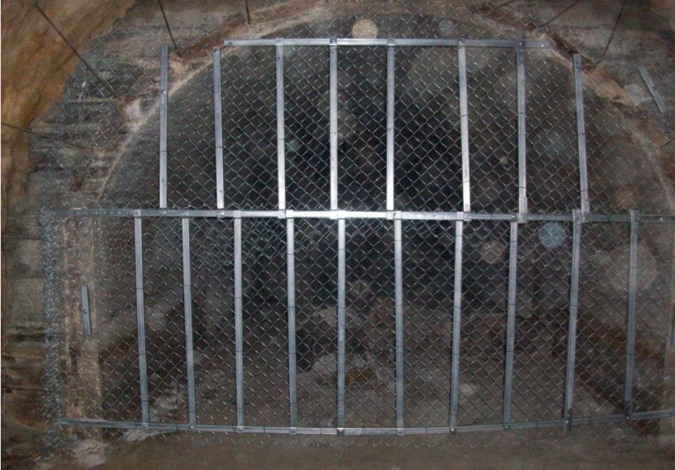
Barrier Wall Construction Completion.
