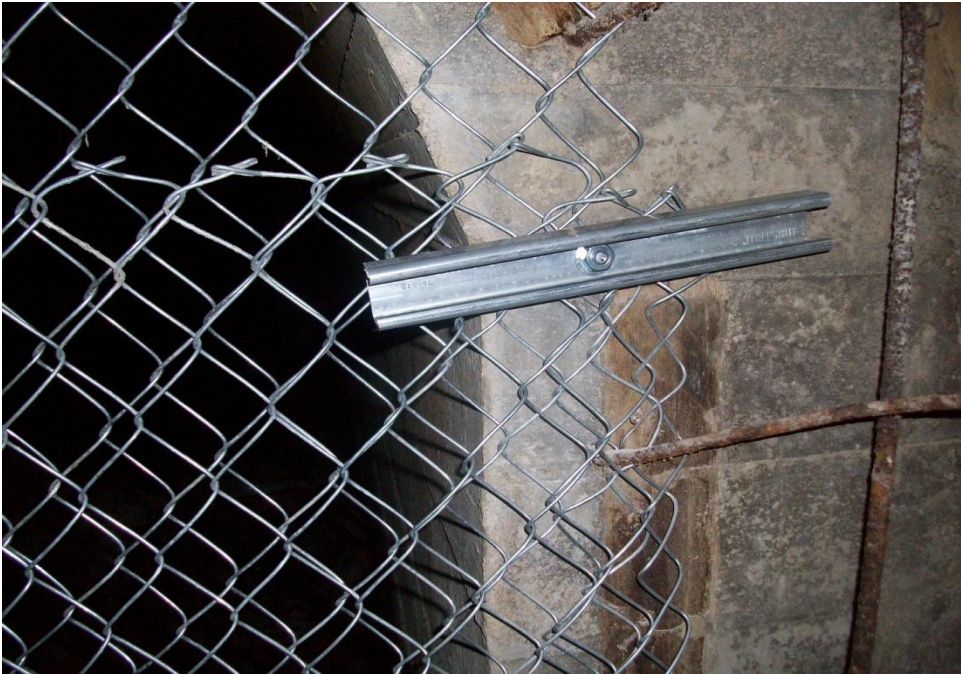
Close-Up of Securing the Chain Link Fencing to the Concrete Wall.
