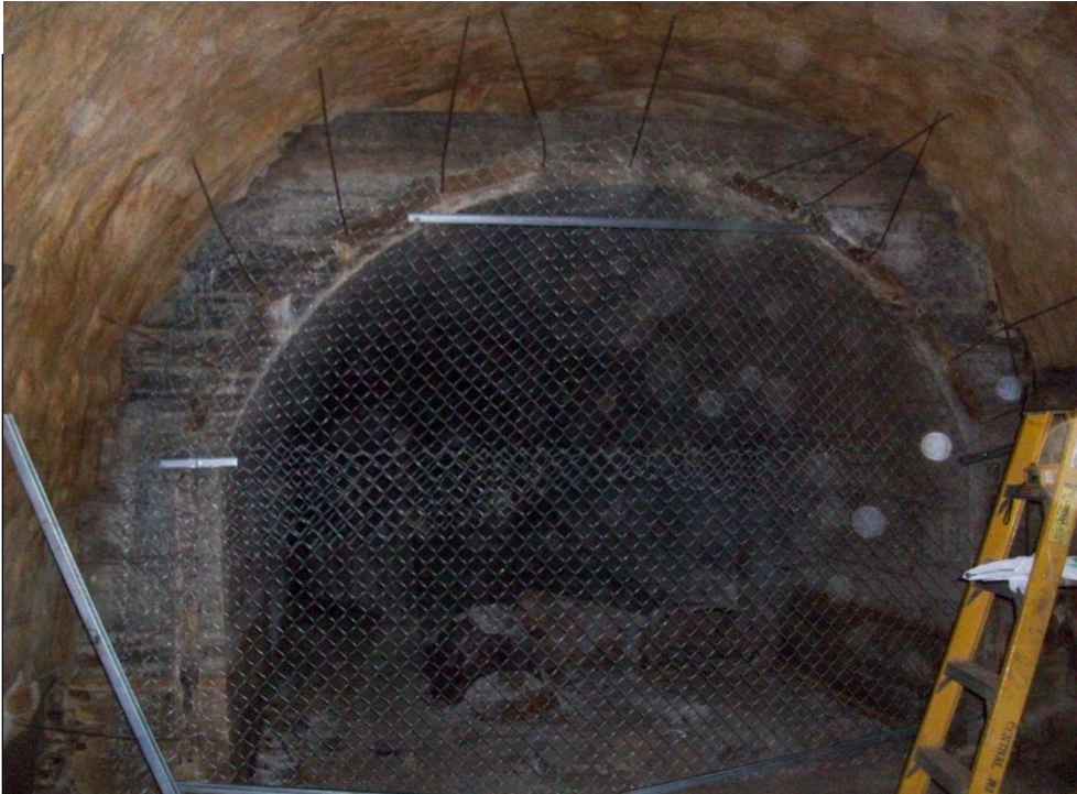
Securing the Chain Link Fencing to the Concrete Wall.
