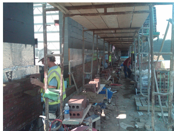
Finish brick on the Community Room.
