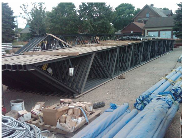
Steel bar-joists for the roof.
