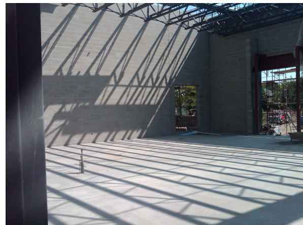
Community room waiting for a roof.
