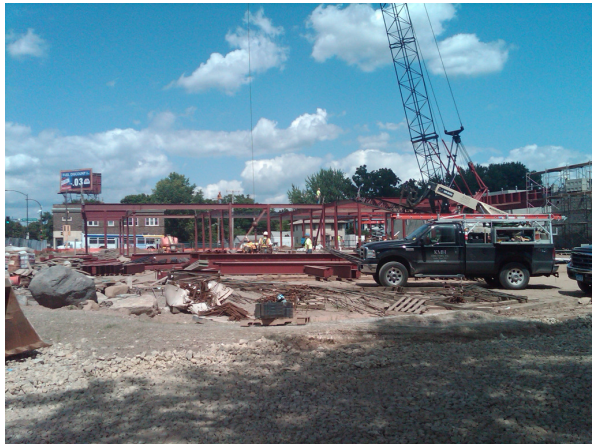
Serious construction activities.
