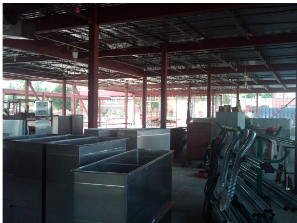
More ductwork and piping supplies.
