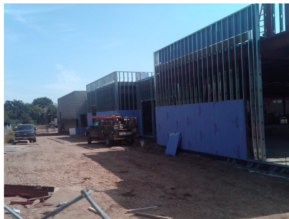
North wall of library and gymnasium.
