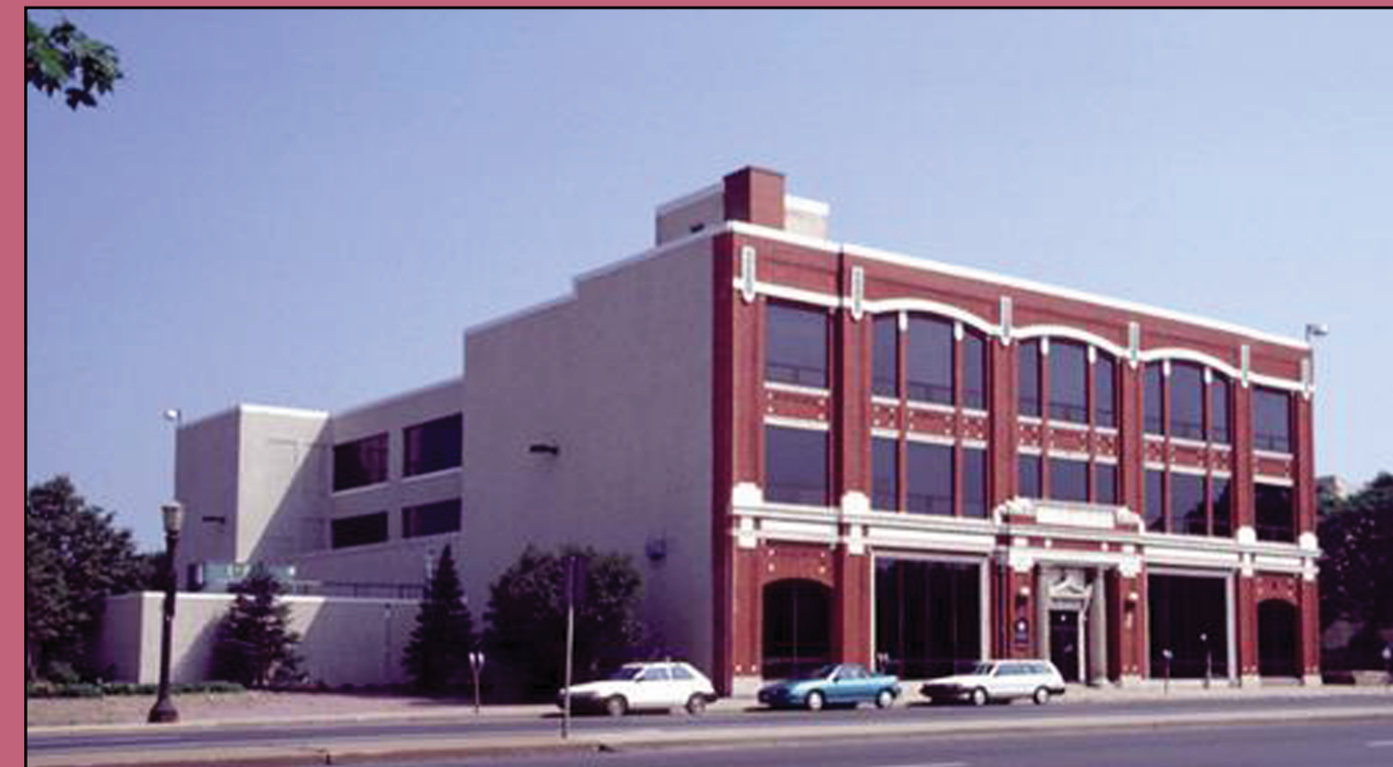
FIGURE 1.4 - Historic Ford Building
