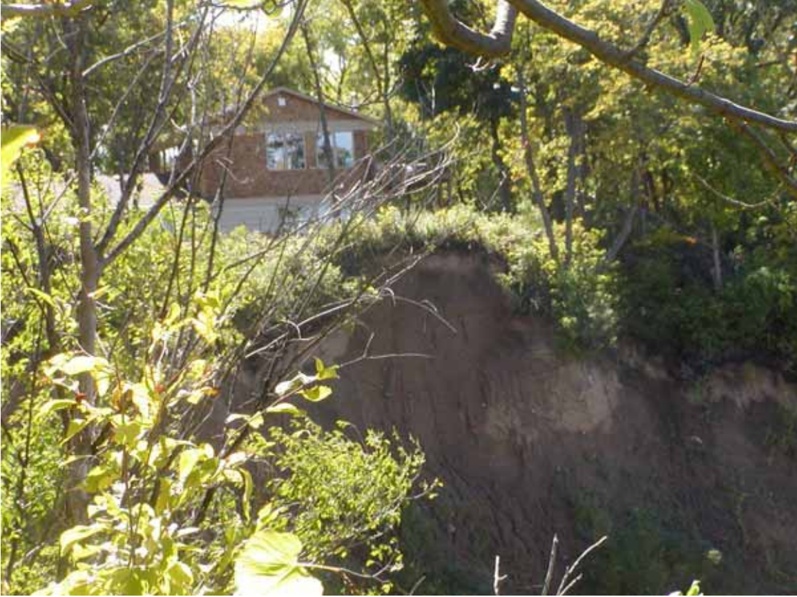
The sheer face of this former clay pit wall occurs in close proximity to a residential home.
