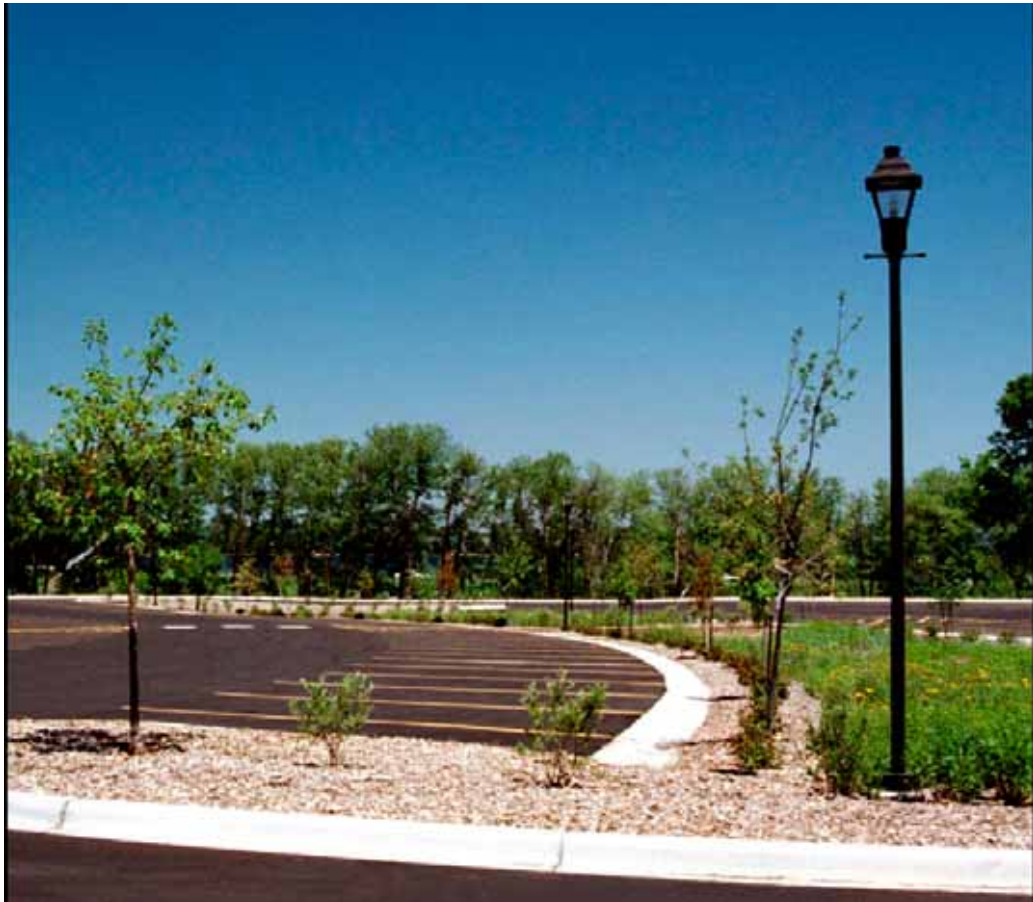
Rain gardens, such as this one at the University of Minnesota Landscape Arboretum offer opportunities to capture and treat stormwater runoff before it reaches surface waters such as lakes and rivers.
