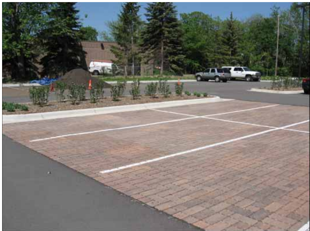
Infiltration features also serve as important opportunities to capture and treat runoff. In this case, permeable pavers also contribute to the aesthetic appeal (Bonestroo headquarters parking lot).
