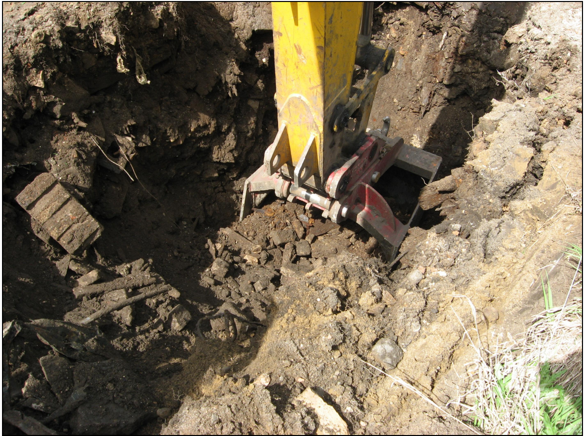
Photograph #5 Subject: Test Pit 2
