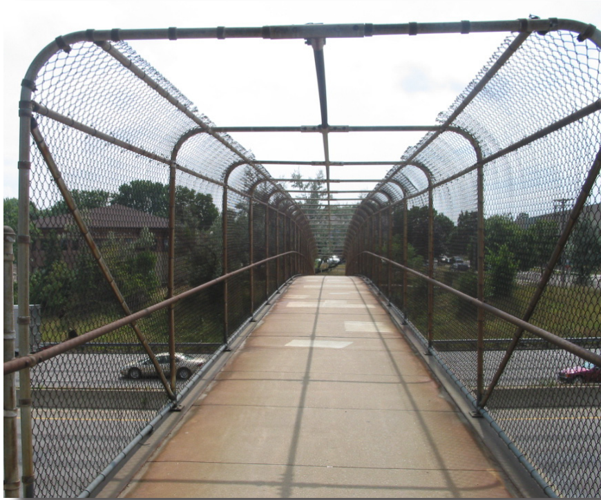
Existing pedestrian bridge over Interstate 94
