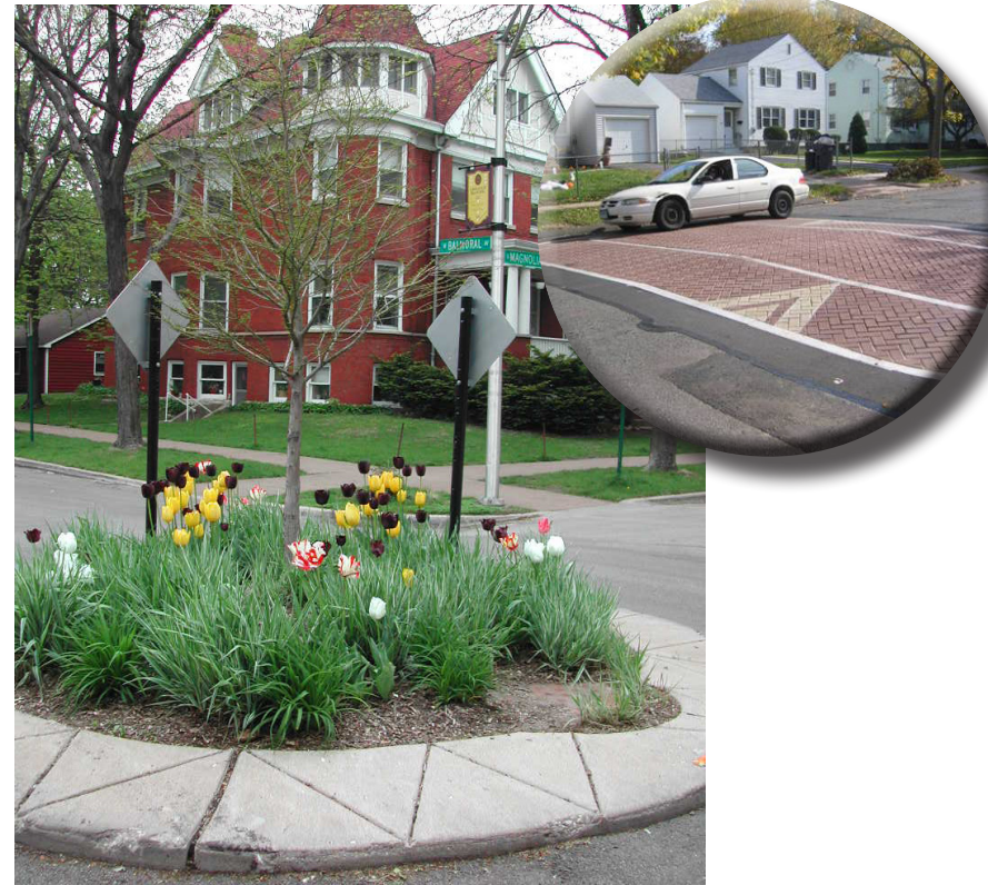
Neighborhood traffic circle in Chicago, and an example of a raised crossing
