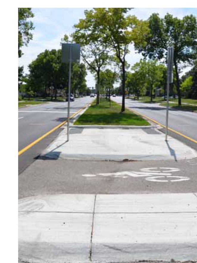
An example of a bicycle / pedestrian refuge island on the Charles Avenue Bicycle Boulevard
