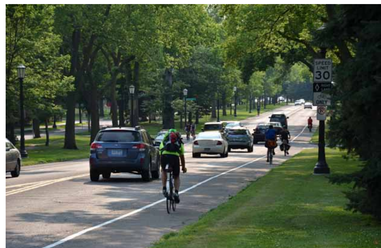
Bike lanes on Summit Avenue directly abutting the curb (no gutter pan)
