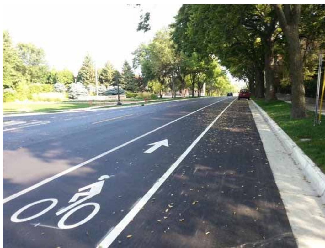
Recent bike lane implementation on Western Avenue with parking maintained on one side of the street
