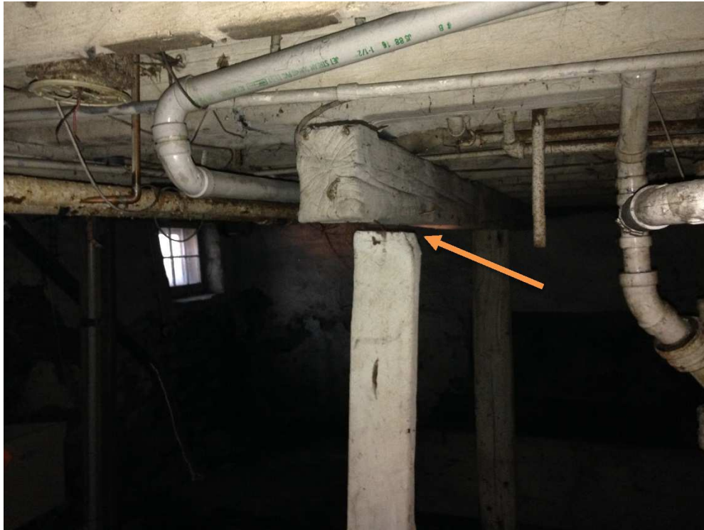
Picture 9 – Beam Above Column in Basement
