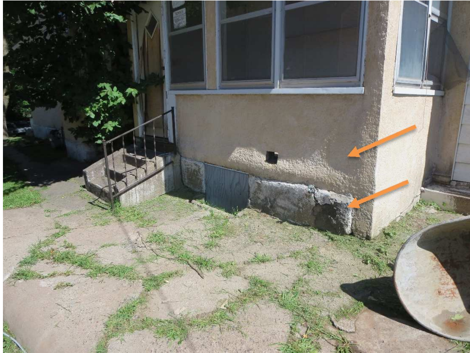
Picture 7 – Water Damage at Southern Foundation Wall
