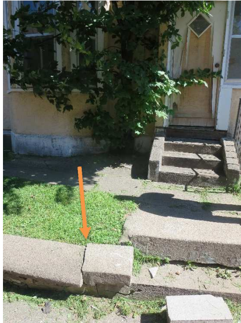
Picture 4 – Crack at South Retaining Wall
