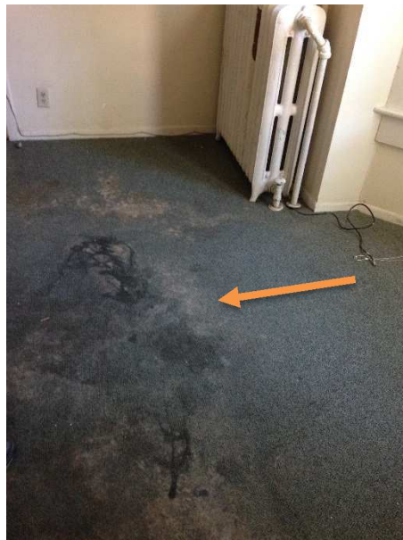
Picture 8 – Water Damage in 2 nd Floor
