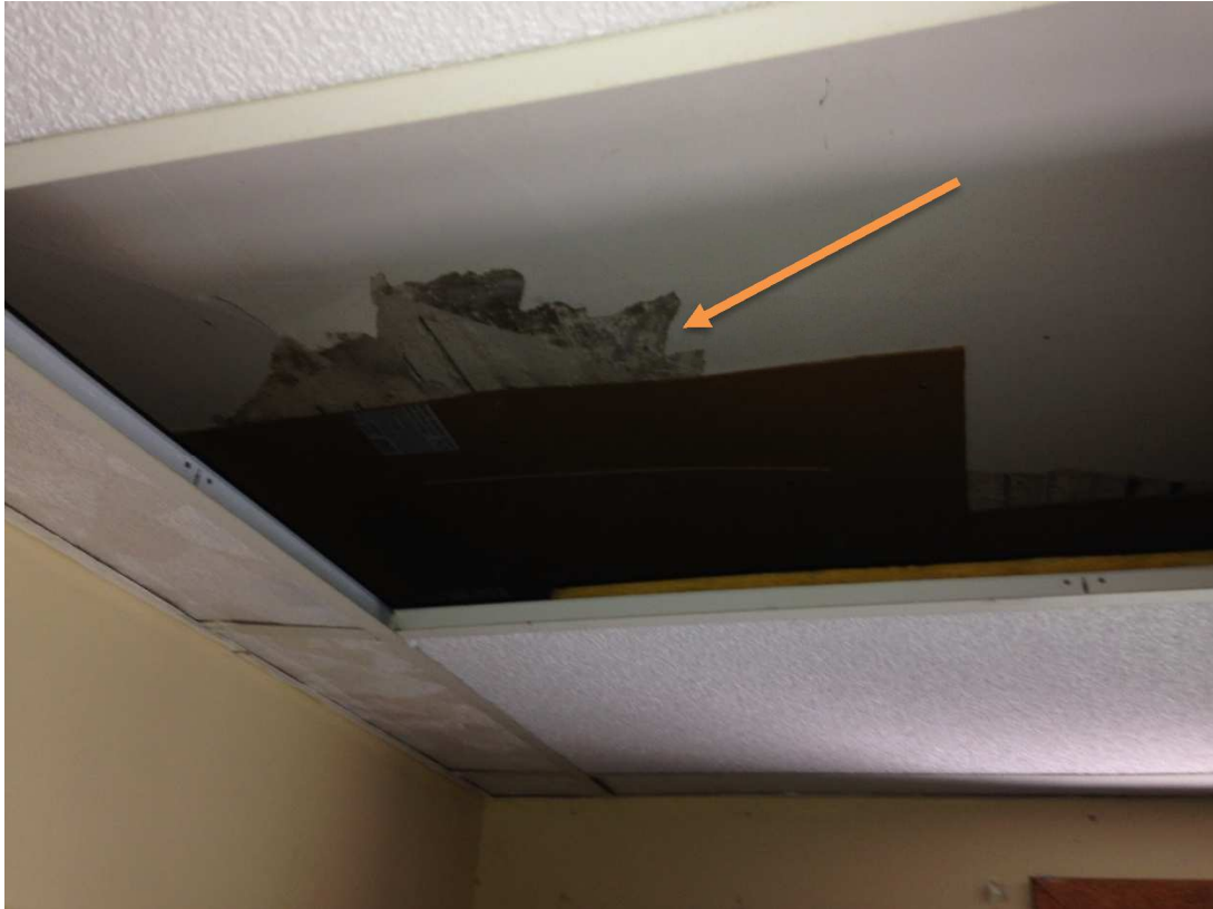
Picture 4 – Water Damage to 2 nd Floor Ceiling
