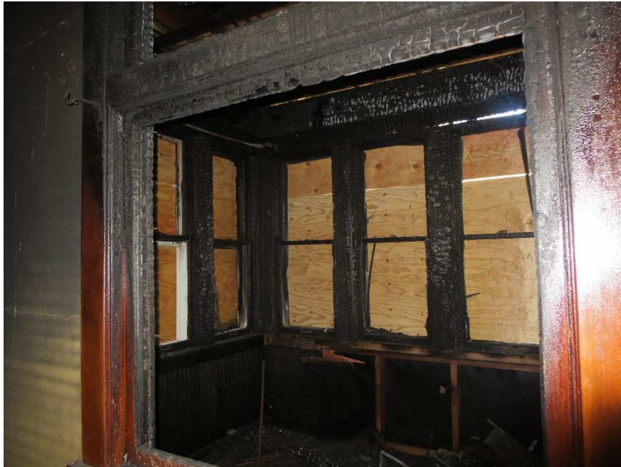
Picture 2 – Front Porch Fire Damage
