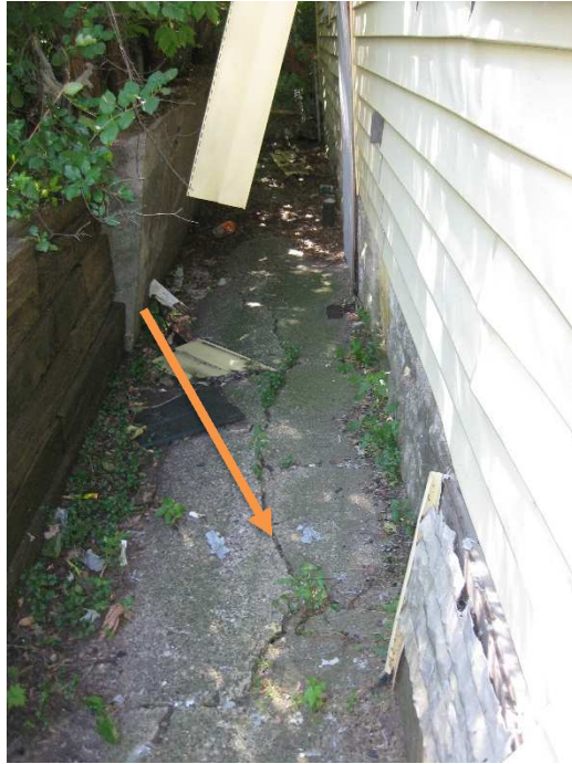
Picture 4 – Crack in Sidewalk at Northeast Corner
