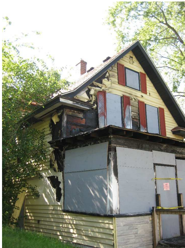
Picture 3 – Fire Damage, Northeast Elevation
