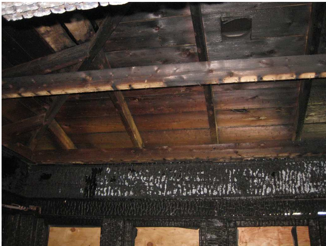
Picture 1 – Front Porch Fire Damage
