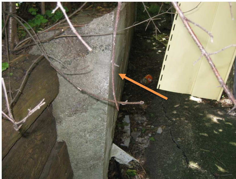
Picture 12 – Rotated Foundation Wall
