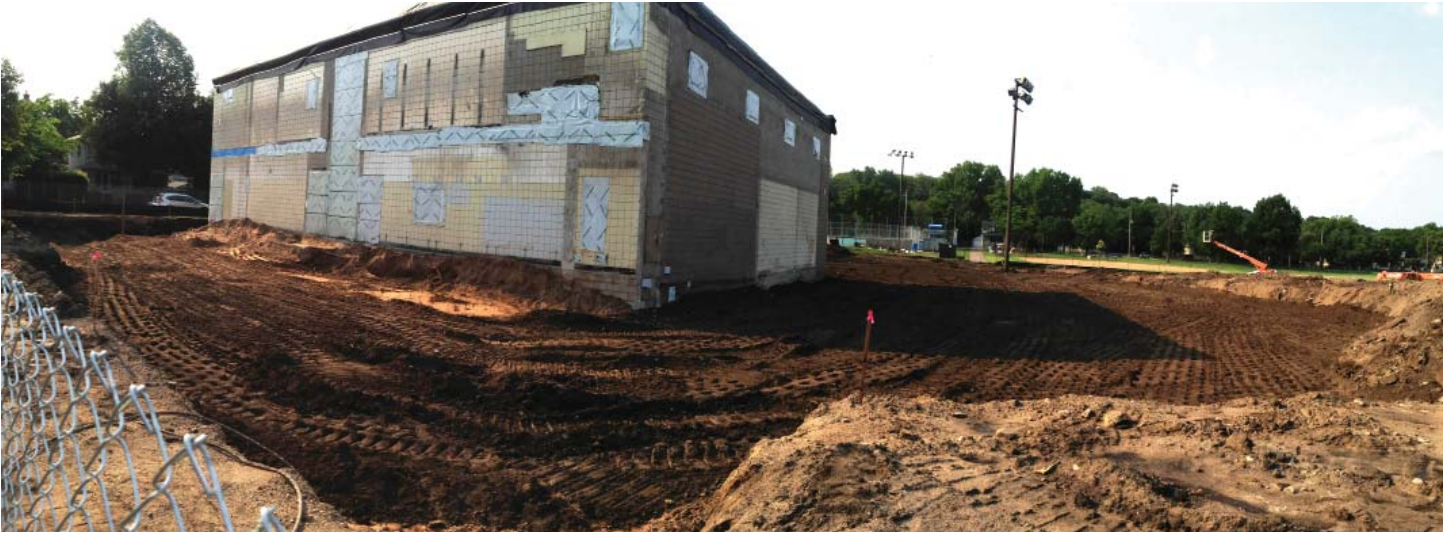
5. Excavations in progress for new foundations and footings (6/8/15)
