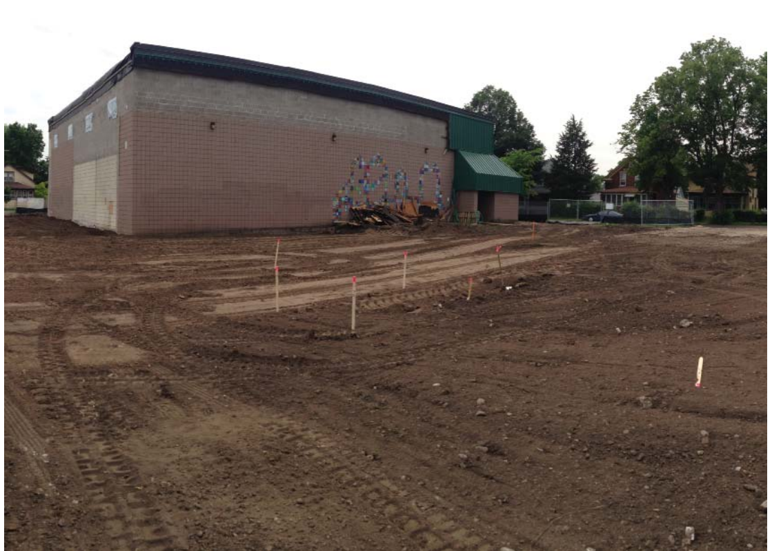
6 and 7. Staking locations for footings and foundations (6/10/15)
