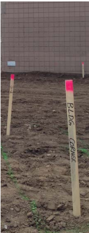
6 and 7. Staking locations for footings and foundations (6/10/15)
