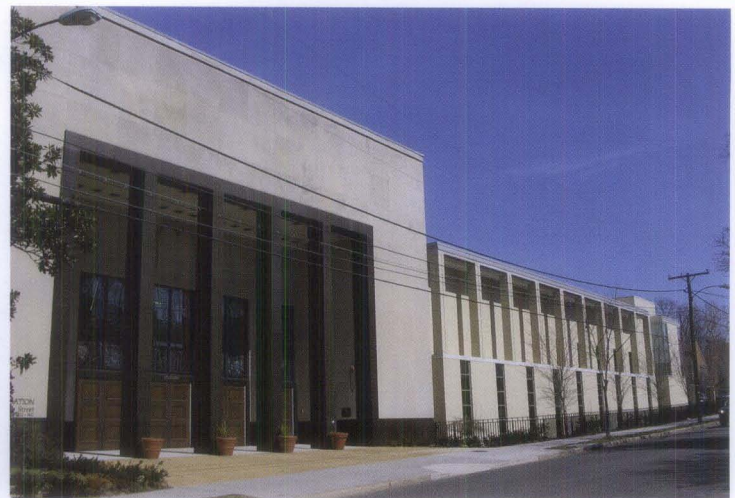
Figure 12. This 1954 synagogue (left) is accessed through a monumental entrance to the right. The new education wing (far right) added to it features the same vertical elements and color and, even though it is quite large, its smaller scale and height ensure that it is secondary to the historic resource.
