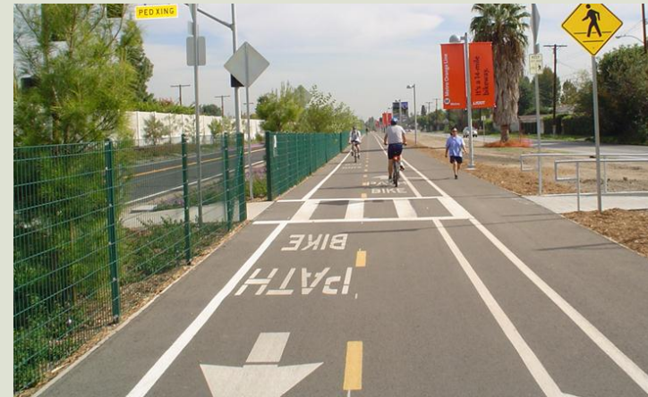
BRT Metro Orange Line – Los Angeles
