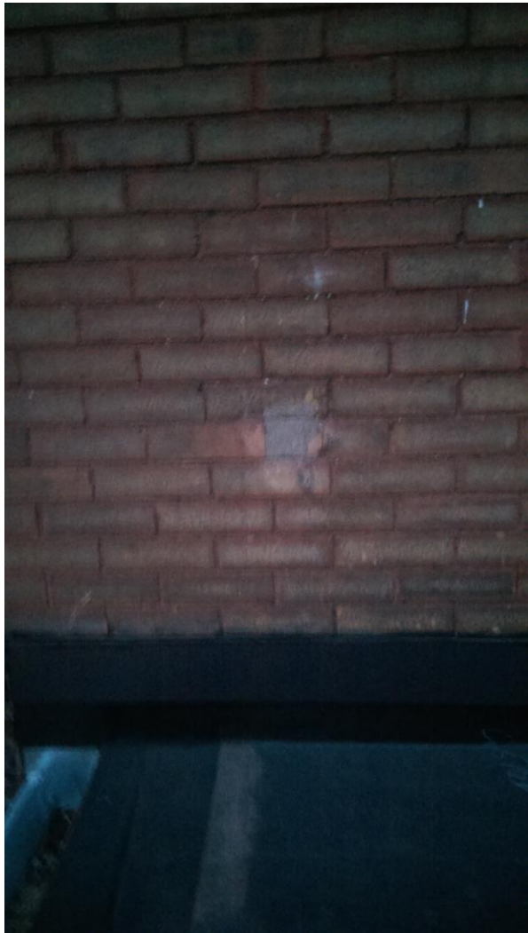
Wider view of west side patch from original railing
