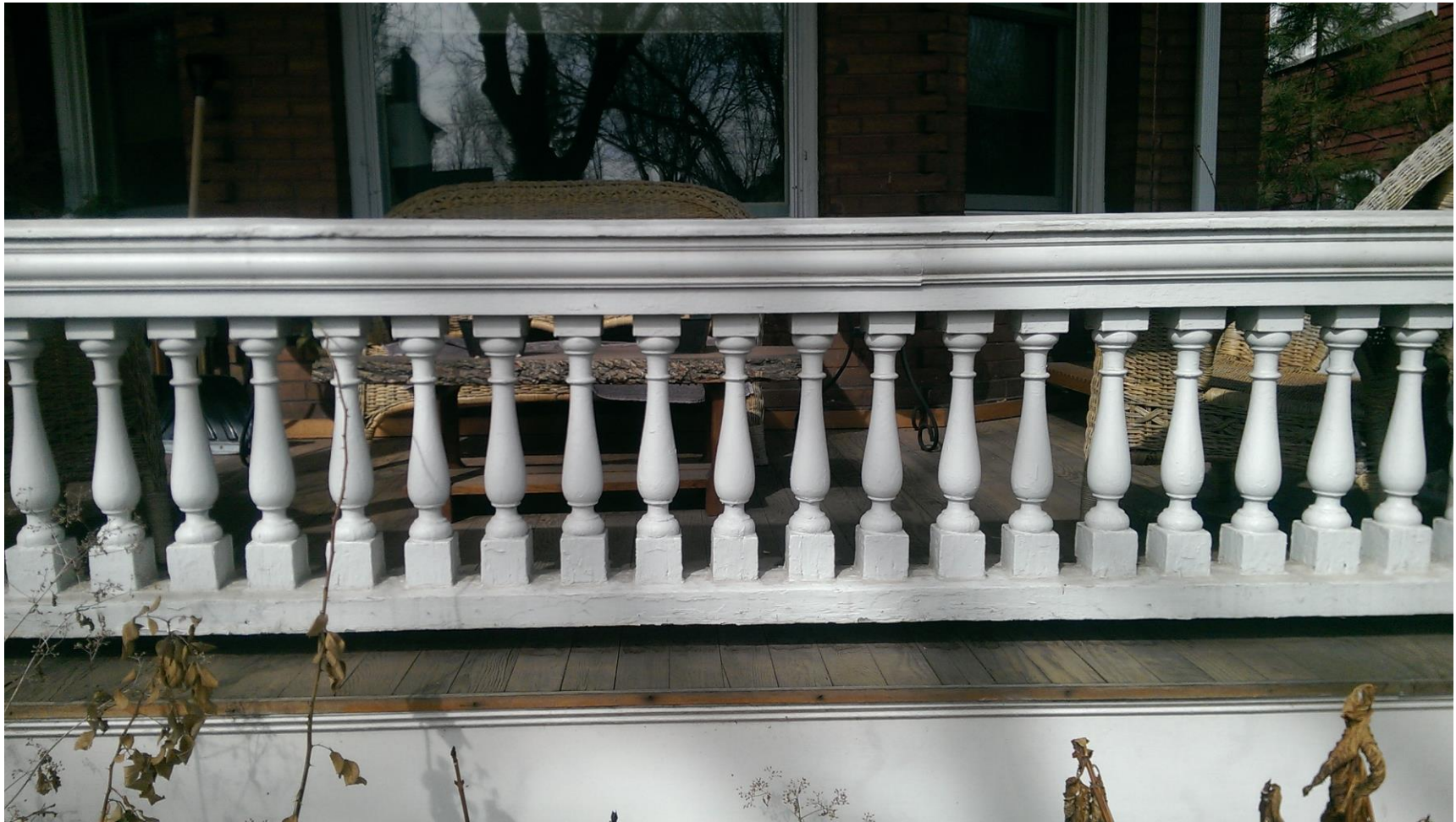
Lower-level balustrades close-up
