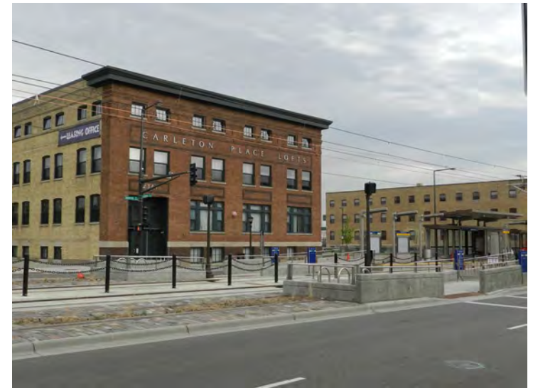
Raymond Avenue Light Rail Station
