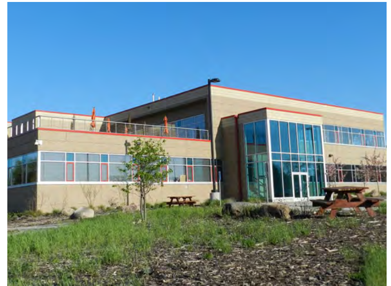
New industrial development at Pierce Butler and Grotto Street
