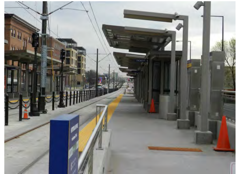
Raymond Avenue Green Line Light Rail Station
