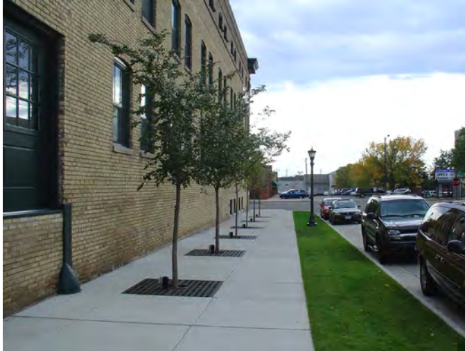
New sidewalk and streetscape on Carleton Street
