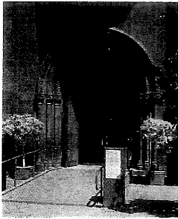
Figure 12. The Smithsonian Institution installed a temporary ramp on its visitor's center to allow adequate time to design an appropriate permanent ramp. Photo: Thomas Jester.
