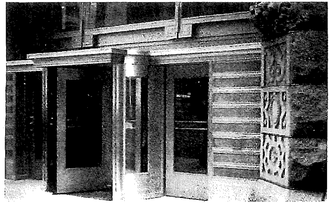
Figure 16. During the rehabilitation of the Rookery in Chicago, the original entrance was modified to create an accessible entrance. Two revolving doors were replaced with a new one flanked by new doors, one of which is operated with a push-plate door opener. Photo: Thomas Jester.
