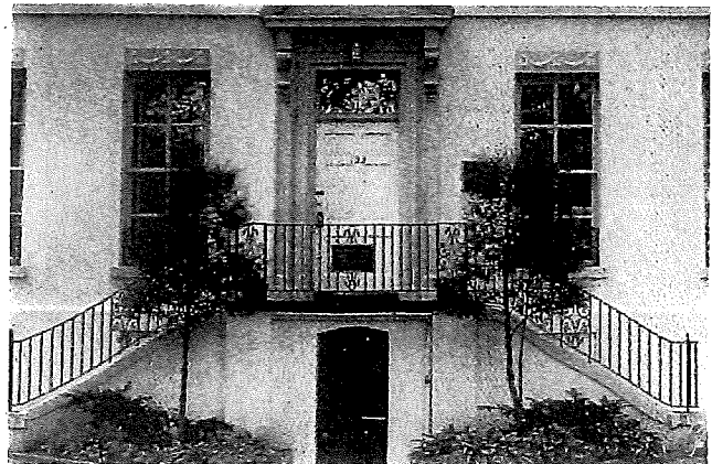
Figure 1. It is important to identify the materials, features, and spaces that should be preserved when planning accessibility modifications. These may include stairs, railings, doors, and door surrounds. Photo: National Park Service files.
