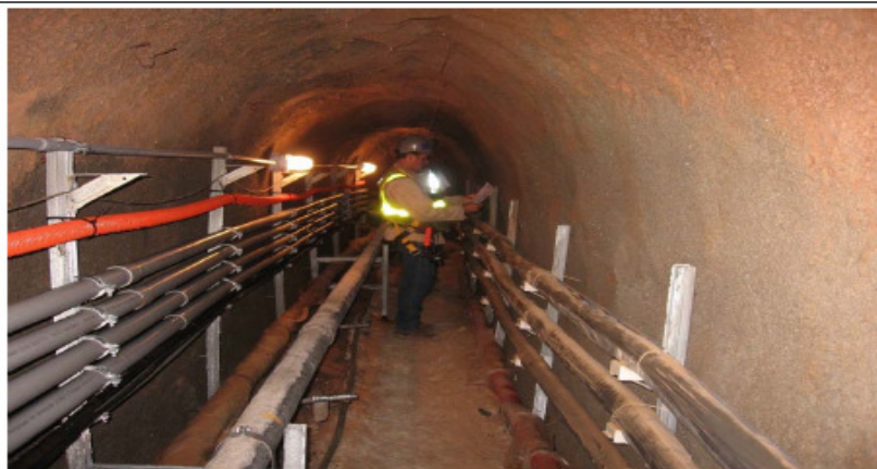
Picture No. 49 – Utility / Cable tunnel near end
