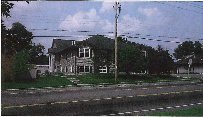
Subject Property: From East
