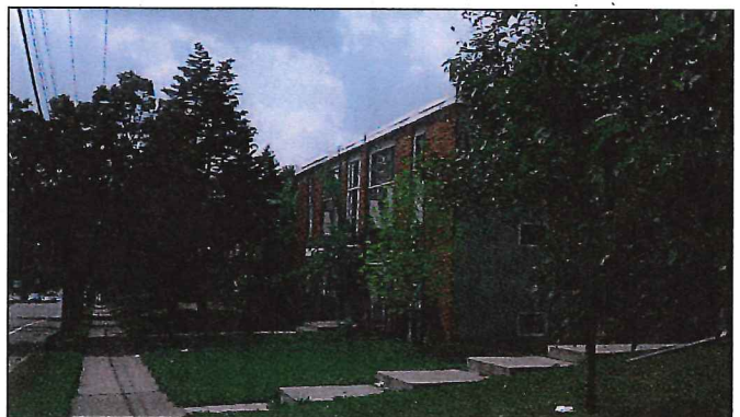
South of subject property
