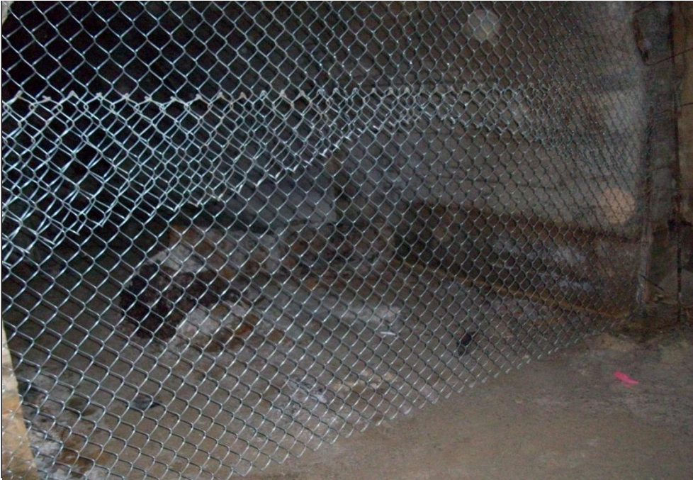
Chain Link Fencing Installation.
