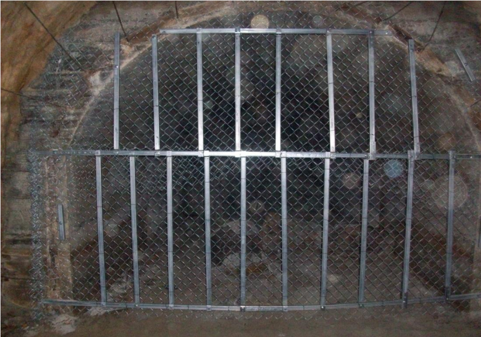
Barrier Wall Construction Completion.
