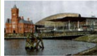
Balance of historic and contemporary roof line treatments.
