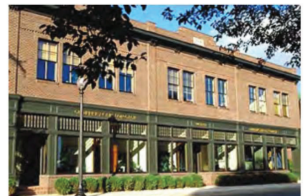
Examples of effective differentiation between ground floor and upper levels
