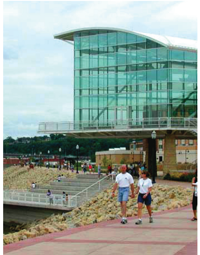
Burying the old concrete flood walls as part of the Mississippi Riverwalk allowed new facilities such as the Grand River Event and Conference Center to fully embrace the riverfront
