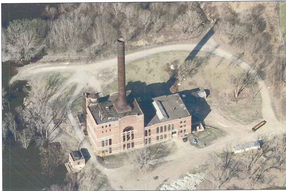
Figure 8. Island Station, looking northwest, 2012. (Bing)
