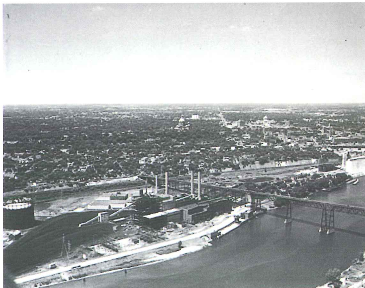
Figure 14. NSP High Bridge Plant (1924), in 1958, looking northeast.
