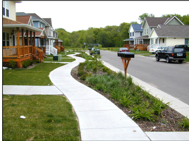
Rainwater gardens can be fit into small and irregular shapes, such as this Habitat for Humanity development. Project by Barr.
