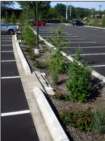
Rainwater gardens in Minnetonka City Hall's parking lots treat stormwater. Project by Barr.
