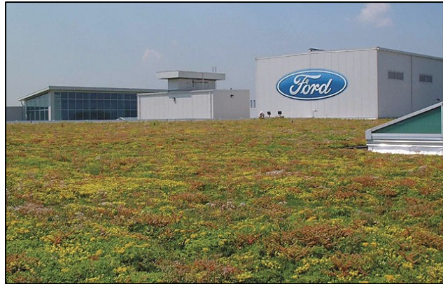
Ford's Rouge Plant in Dearborn, Michigan has the world's largest green roof. Photo from www.greenroofs.org
