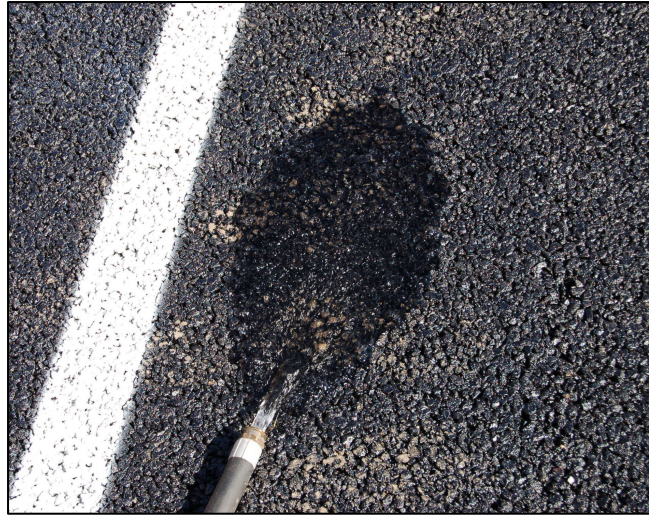
Porous Pavement at Ramsey Washington Metro Watershed District's new offices. Project by Barr.
