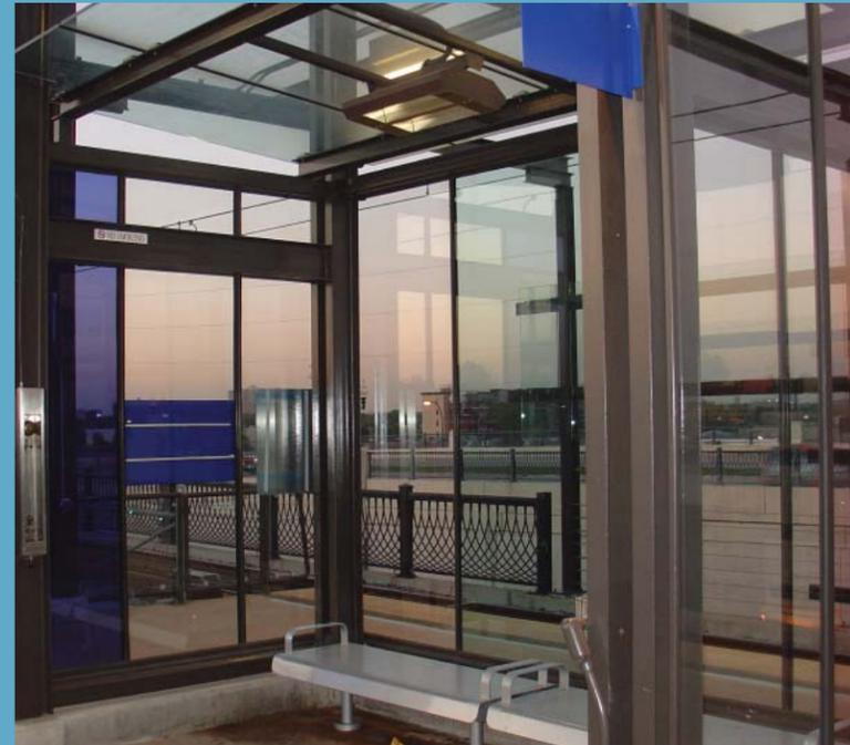
This shelter on the Hiawatha Line provides for passenger comfort with seating and an overhead heater for the winter months.
