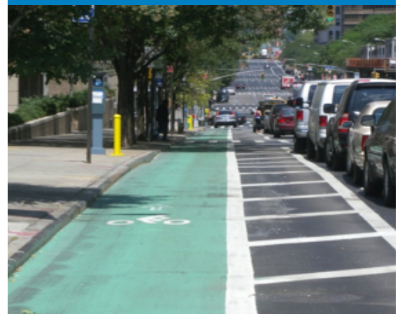
A one-way cycle track protected by a parking lane and buffer and showing optional green paint
