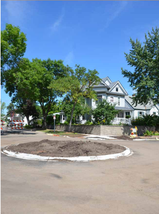
Construction of the Griggs Ave Bicycle Boulevard
