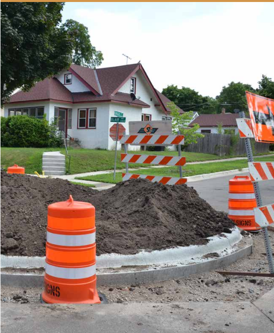
Griggs bicycle boulevard under construction
