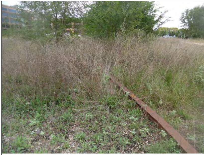
Photo 12: Railroad rail on ground surface, not in alignment with known spur locations.
