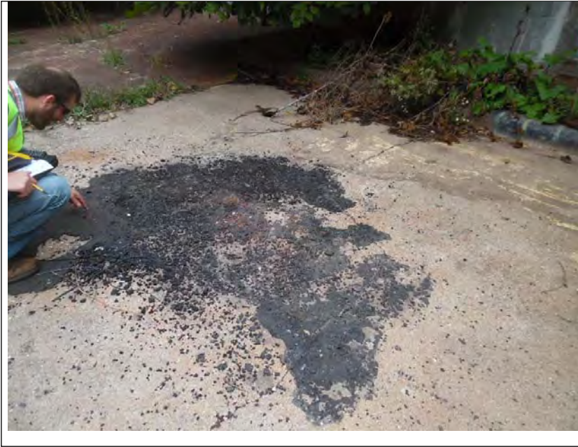
Photo 9: Burn substance remains west side of remaining building.
