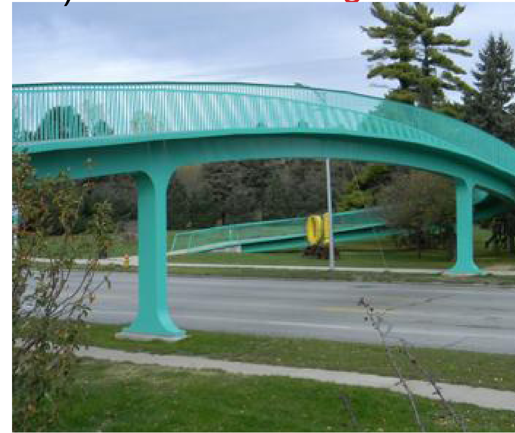
A3) Pedestrian Bridge
