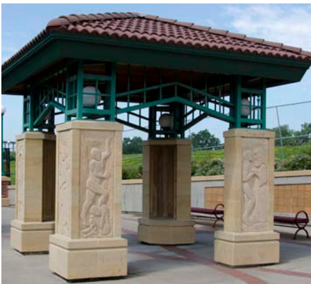
Wayfinding Kiosk at Harriet Island
