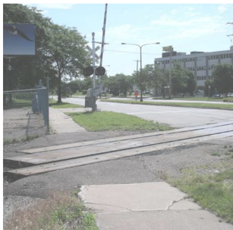
Track Crossing Plato Blvd. & Starkey St.
