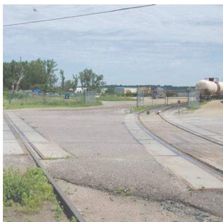
Track Crossings at Barge Channel Rd.
