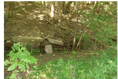
Existing Marina Demolition Site
