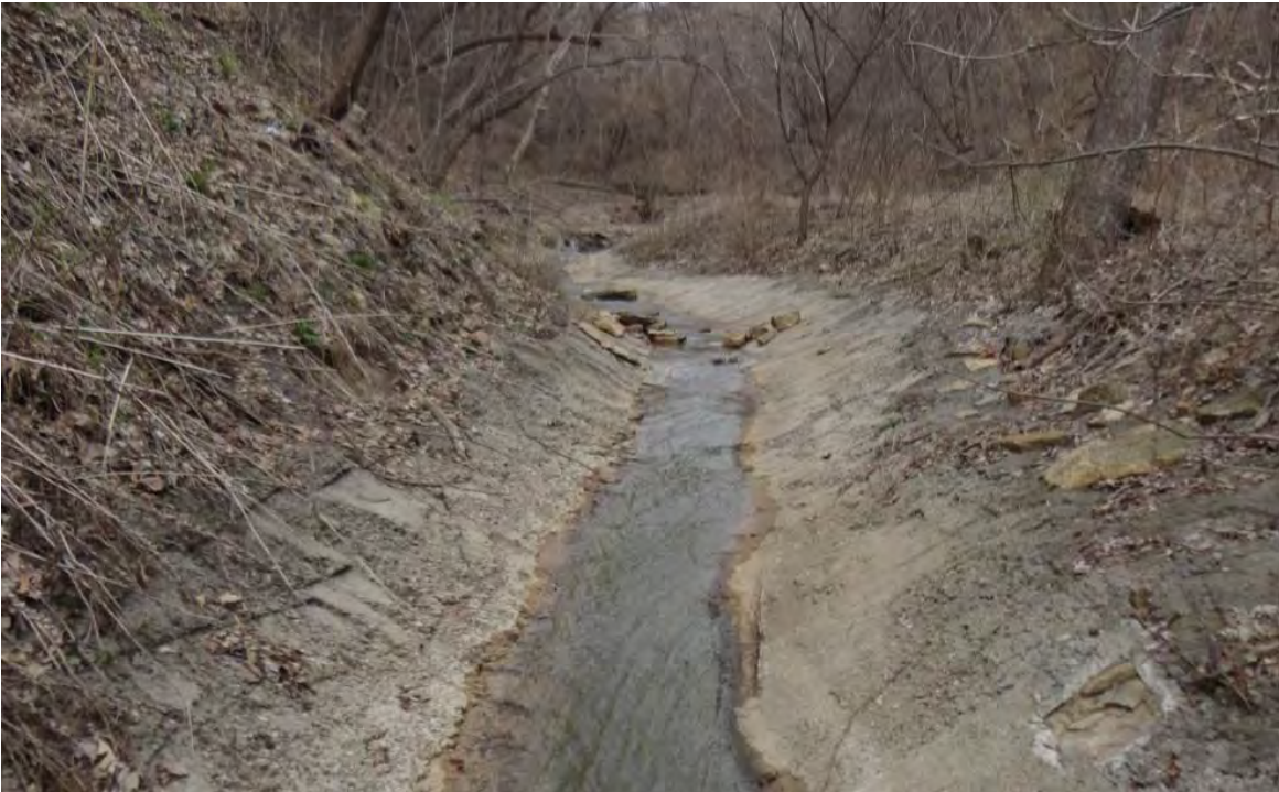
Figure 21: Looking upstream at The Chute along the base of bluff near Station 11+00 – 12+50
