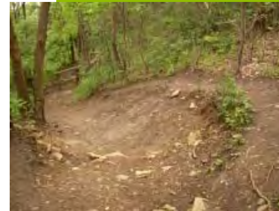
Sloped and eroded trail, where wide stairs are recommended.
