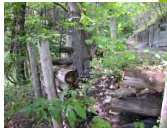
Severely eroded promontory.
