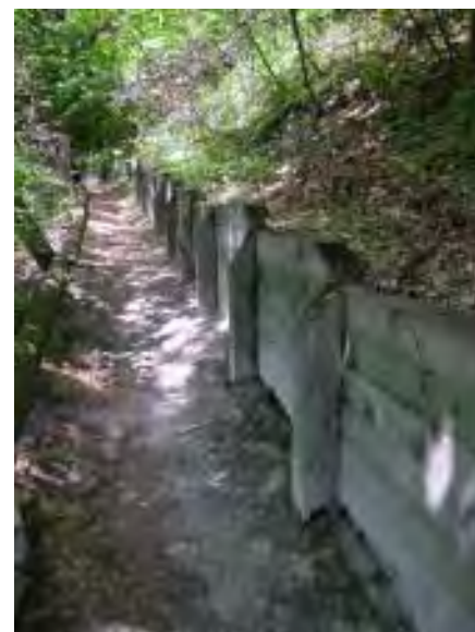
Most recent, sturdy timber wall.
