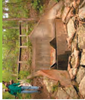
Large storm water outlet structure, an opportunity for interpretation.
