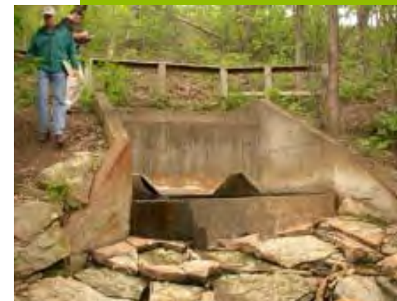
Large storm water outlet structure, an opportunity for interpretation.
