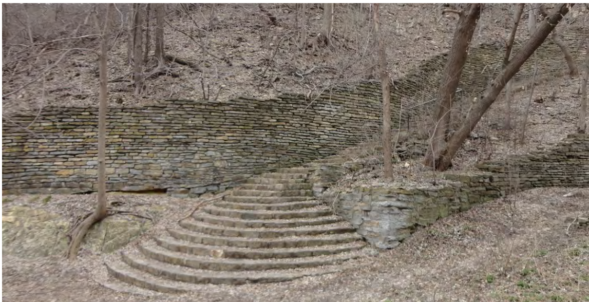
Figure 8: WPA era walls and grand staircase along the eastern edge of Hidden Falls Ravine
