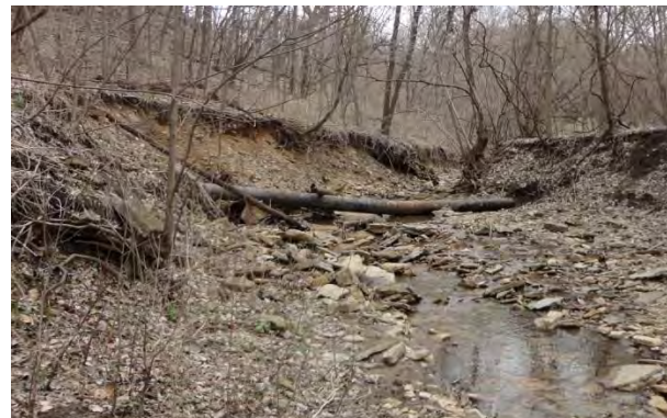
Figure 42: Pipe to be removed.
