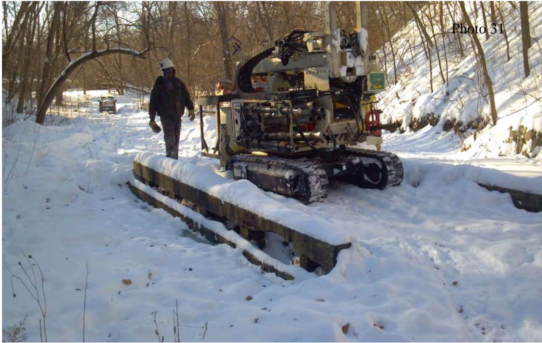
Geo Probe on Re-enforced Bridge
