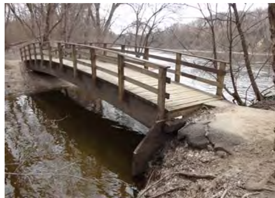
Figure 12: Bridge across Hidden Falls Creek at the Mississippi River
