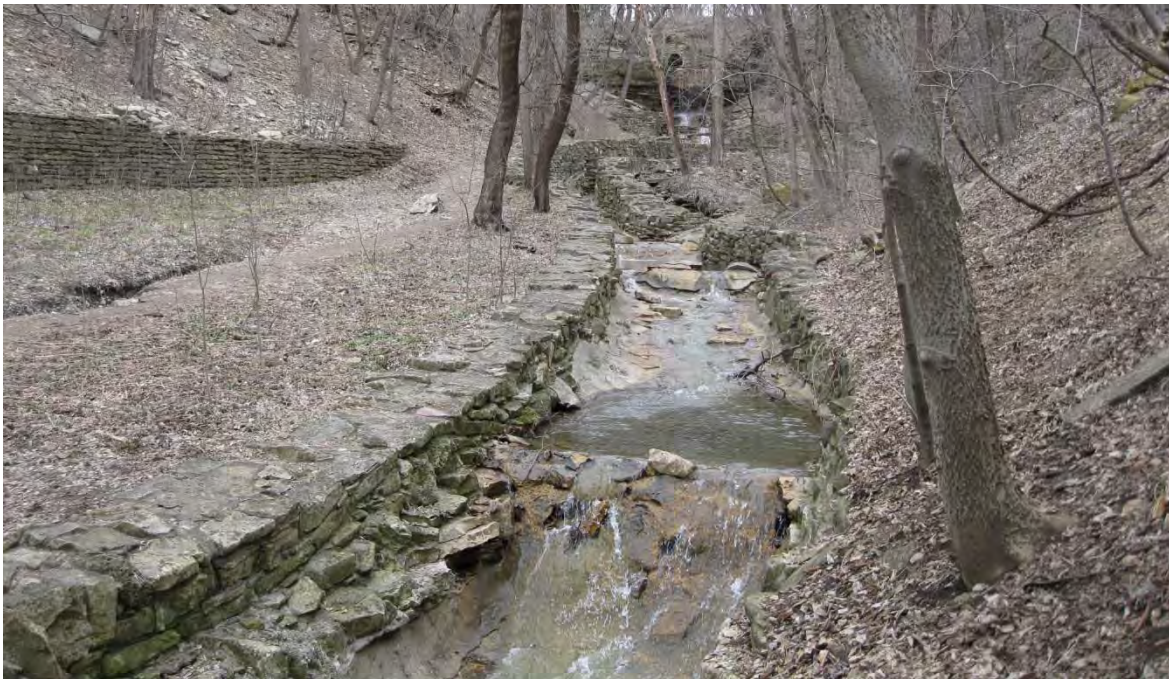
Figure 28: Existing step pool reach at Hidden Falls Creek
