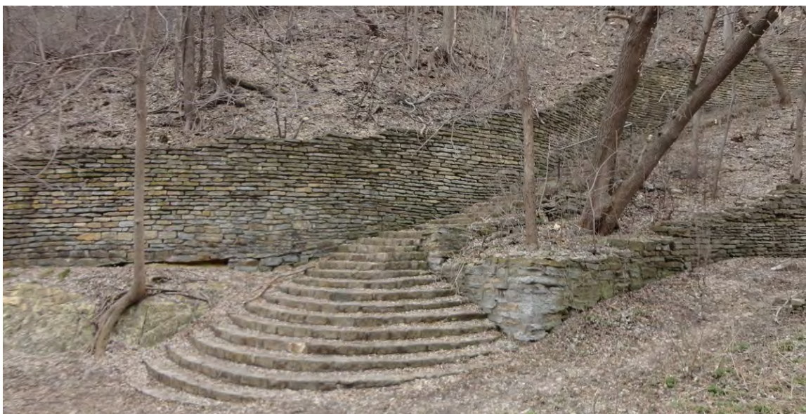
Figure 8: WPA era walls and grand staircase along the eastern edge of Hidden Falls Ravine
