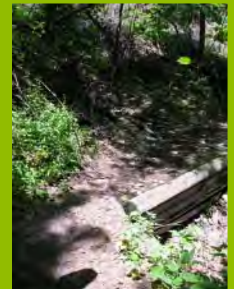
Water on trail, gabion's recommended.
