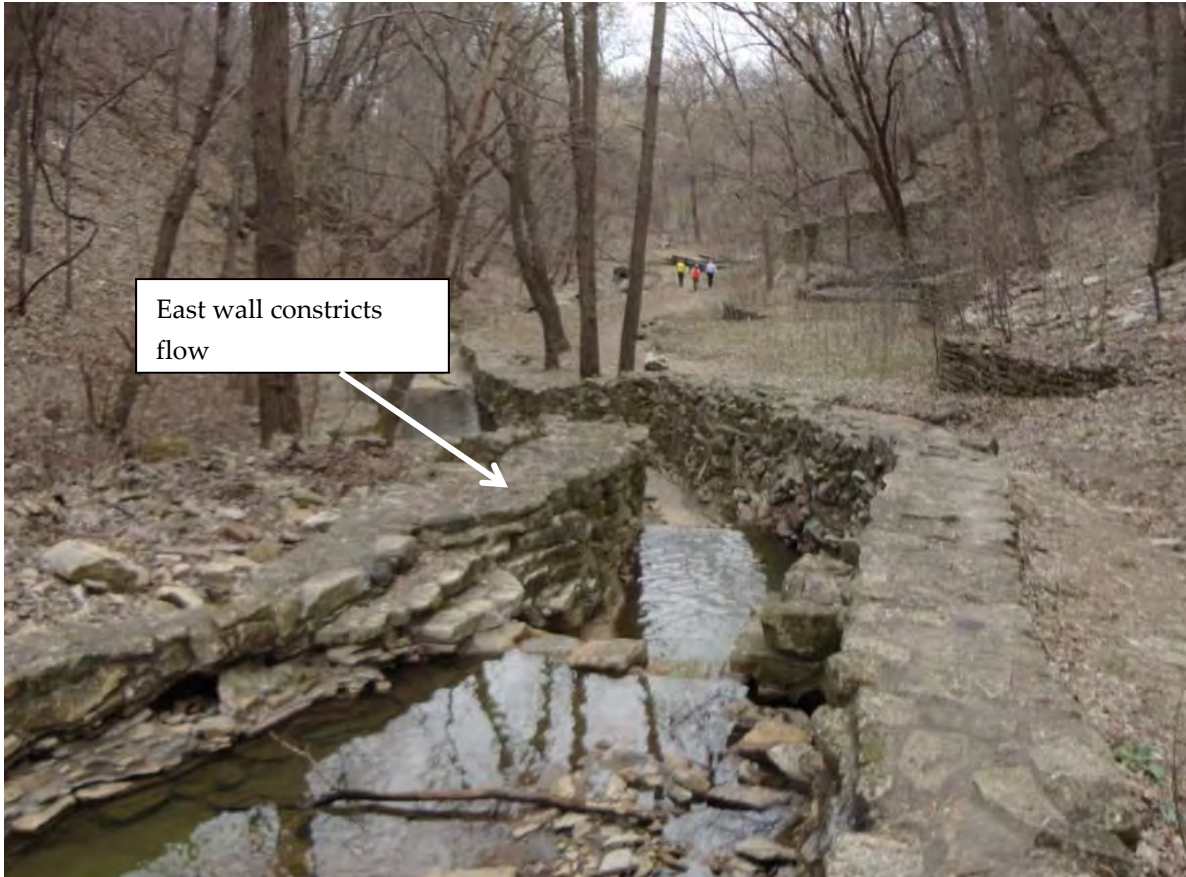
Figure 29: Upper step pool reach showing 1980's era walls considered for removal
