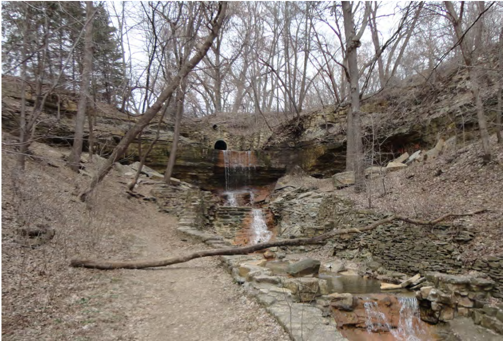
Figure 6: View of Hidden Falls showing the worn and undercut Platteville Limestone caprock, fallen limestone blocks and existing pools and cascades of upper falls
