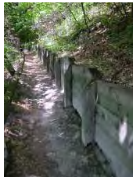
Most recent, sturdy timber wall.
