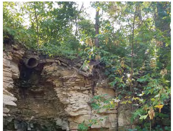
Figure 2.7: Storm drain culvert (polygon 4)
