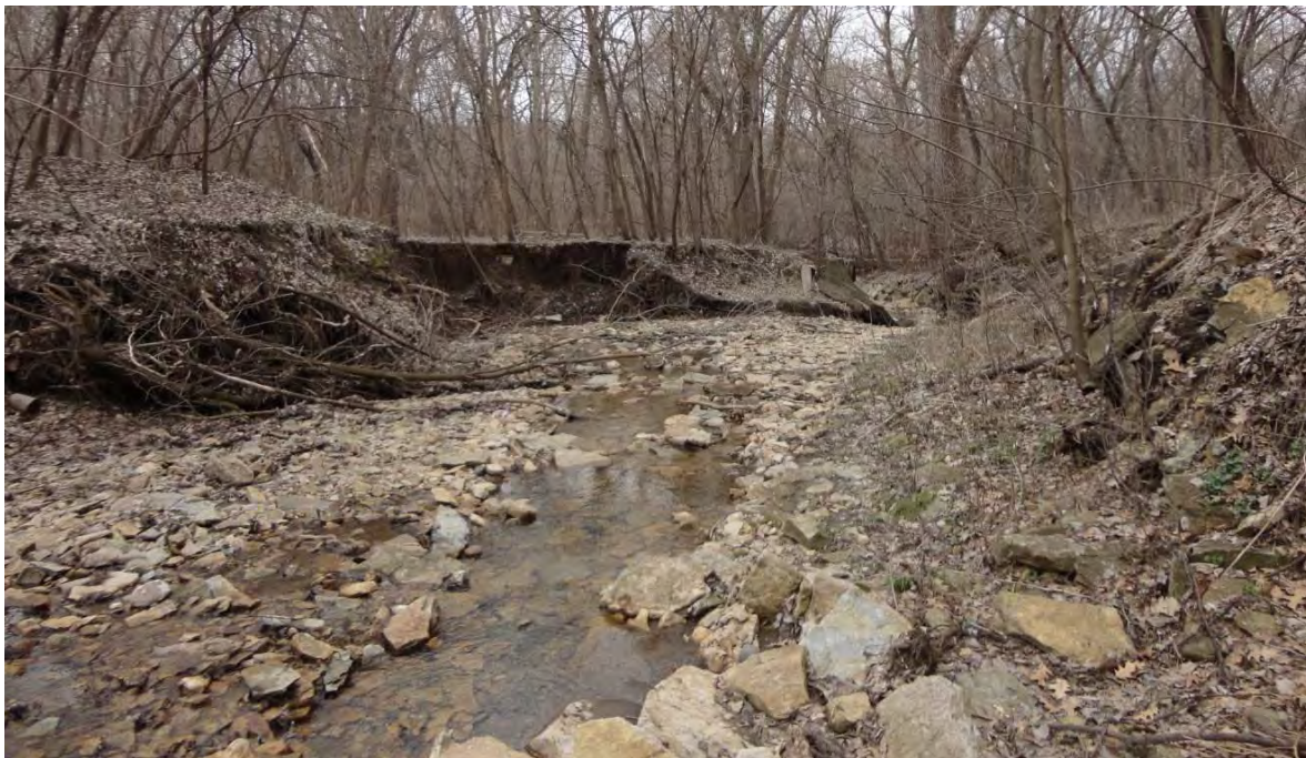
Figure 39: Stable right bank and steep, eroding left bank. Left bank should be graded and stabilized. Channel bed should be reshaped to include a low flow channel and floodplain bench.
