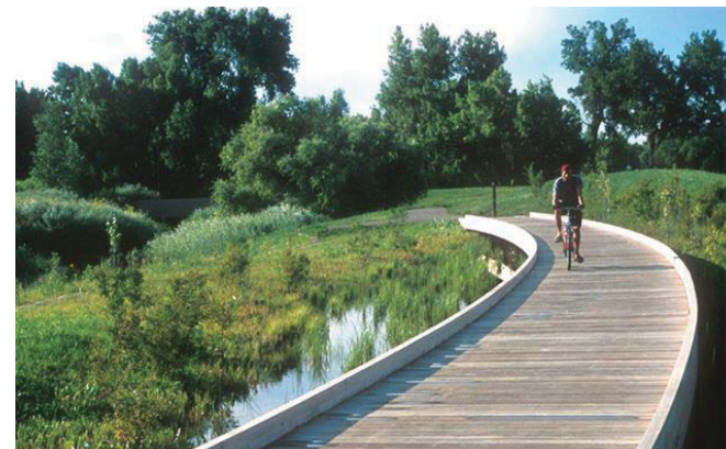
Stormwater treatment areas also provide recreation benefits for the community.
