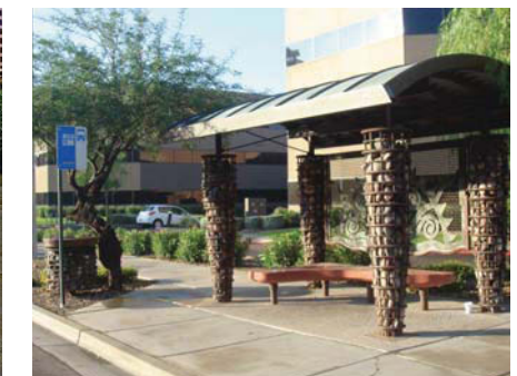
Transit Stops: Unique design, branding and marketing of the river-transit interface is recommended.
