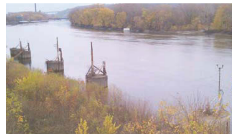
Existing abandoned barge docking facility
