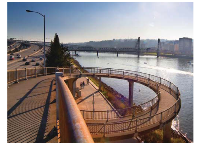
Grade-Separated Crossings: Structures are reserved for roadways with high traffic volumes and speeds, where crossing at a signal is not practical.
