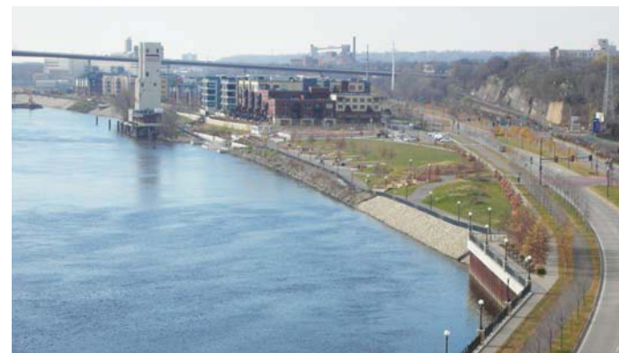
East side River edge at upper landing now: Rip rap banks provide necessary armoring against flooding and commercial River traffic.
