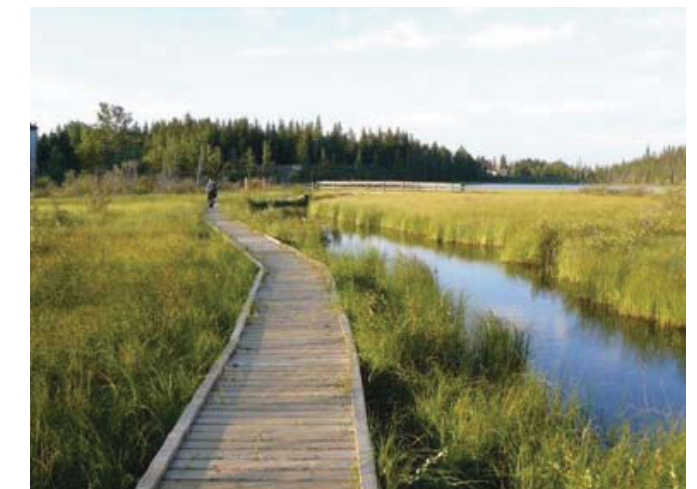
Boardwalks span sensitive environments
