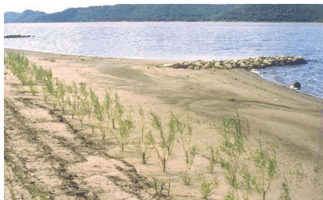
Using rock vanes to restore and stabilize the shoreline enhances riparian habitat.
