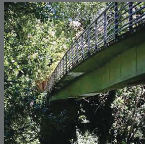
Bridges Over Barriers
