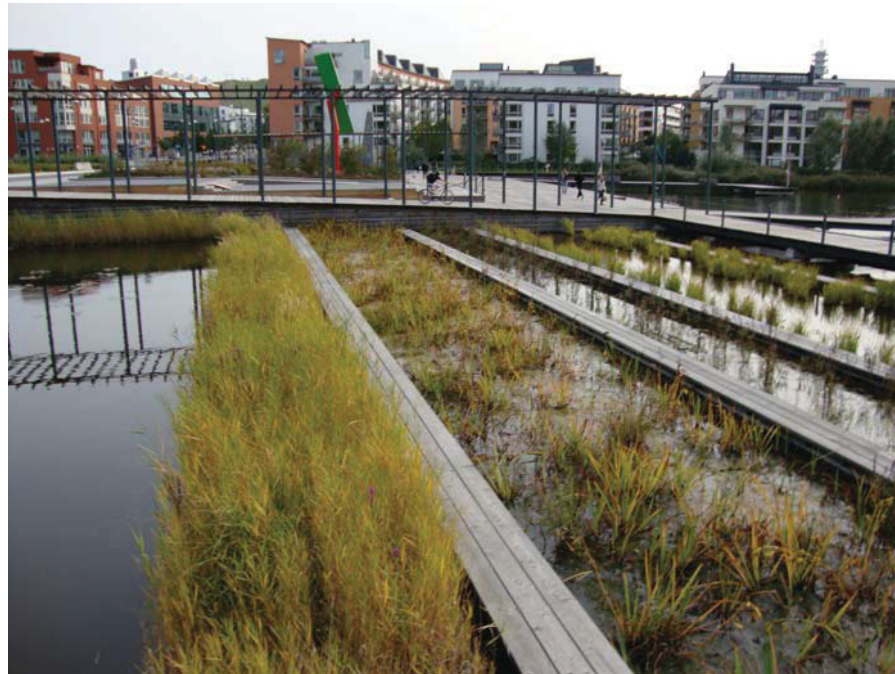
Constructed wetlands improve water quality, erosion control and habitat.
