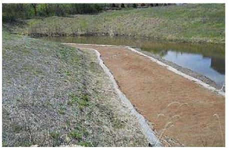
Figure 4: Iron-enhanced sand filter bench at Prior Lake, Minnesota
