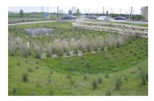
Figure 3: Typical bio-filtration basin
