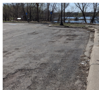
Improve parking lot pavement
