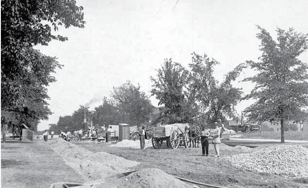
Roadway construction near Summit Avenue and Grotto, 1915 Credit: Minnesota Historical Society
